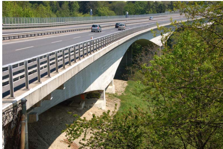
(a) Overall view of the Lutrive Viaducts
