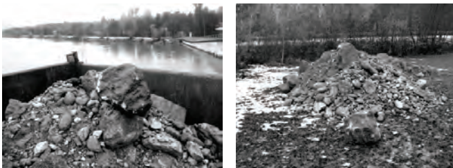
Figure 2. Dredging of sediment accumulated in front of the trash rack, GKW GmbH.
