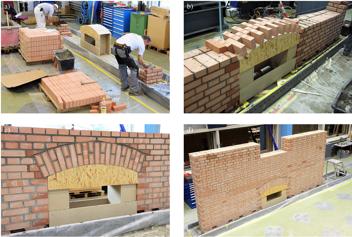
Figure 1.4: Construction of masonry spandrel with arch (TUC).
