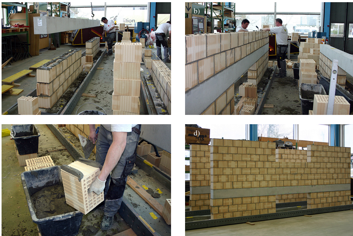
Figure 1.3: Construction of composite spandrels.
