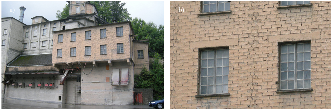
Figure 1.4: URM building with RC lintel serving as a gravel plant in Alt St. Johann (Switzerland): Entire building (a) and lintel detail (b).
