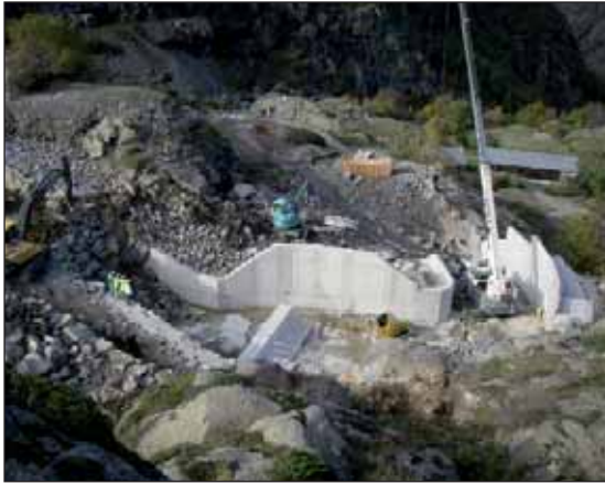
October 2009: The expanding stilling basin and its sidewalls are complete.
