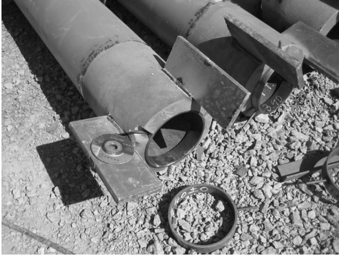
Figure 3. Movable backing ring for on-site assembly
