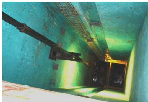
Figure 9: View into the duct of the slide gate chain
