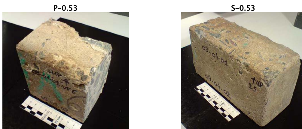
Fig. VI-3. Visual appearance of the field concretes after 19 years under partial immersion (submerged part: bottom of the concrete blocks – exposed part: top of the concrete blocks) in sulfate enriched ground.
