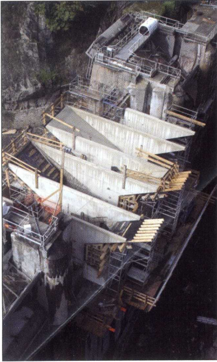
Construction under way at the Saint-Marc PKW and (a, b) vertical walls and (c) the ski jump gutter.
