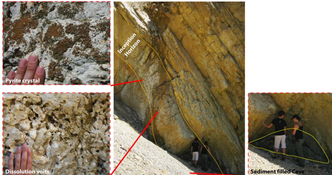
Fig. 3.17: Outcrop of a pyrite rich inception horizon (Court, Switzerland). Left above: locally some not weathered pyrite crystals can be found exposed; Left below: the weathering of the pyrite and the associated production of acid solution produced a very porous looking horizon; Right below: within the horizon a cave conduits cropped out, unfortunately the conduit is filled up with clastic sediments and can not be explored to verify if the conduit follows also in distance the inception horizon.
