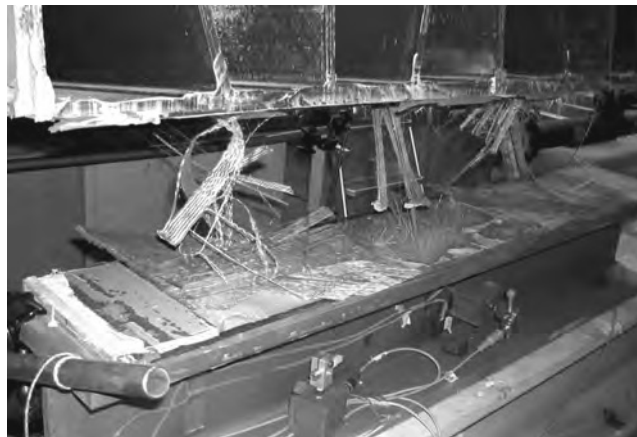
Figure A.16: Failed adhesively-bonded connection (C3-2)
