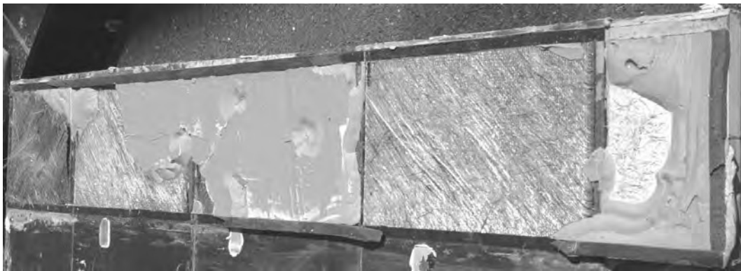
(b) view of deck
