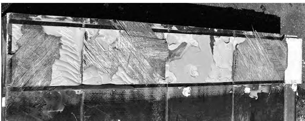
(b) view of deck
