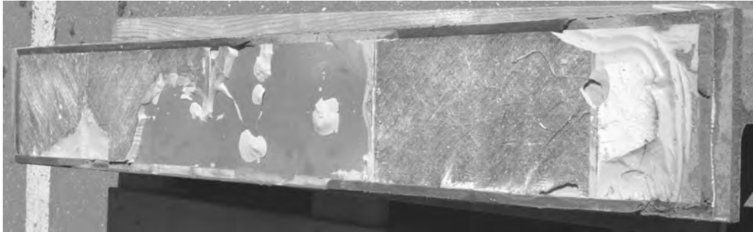
(a) view of girder
