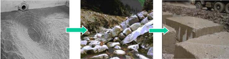
Figure 1: Alluvial bed (left), riprap protection (middle), concrete prisms (right)
