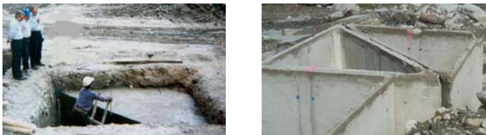
Figure 12: Prisms construction methods, without using sides' formwork and reinforcement (left), precast formwork filled with mass concrete (right)
