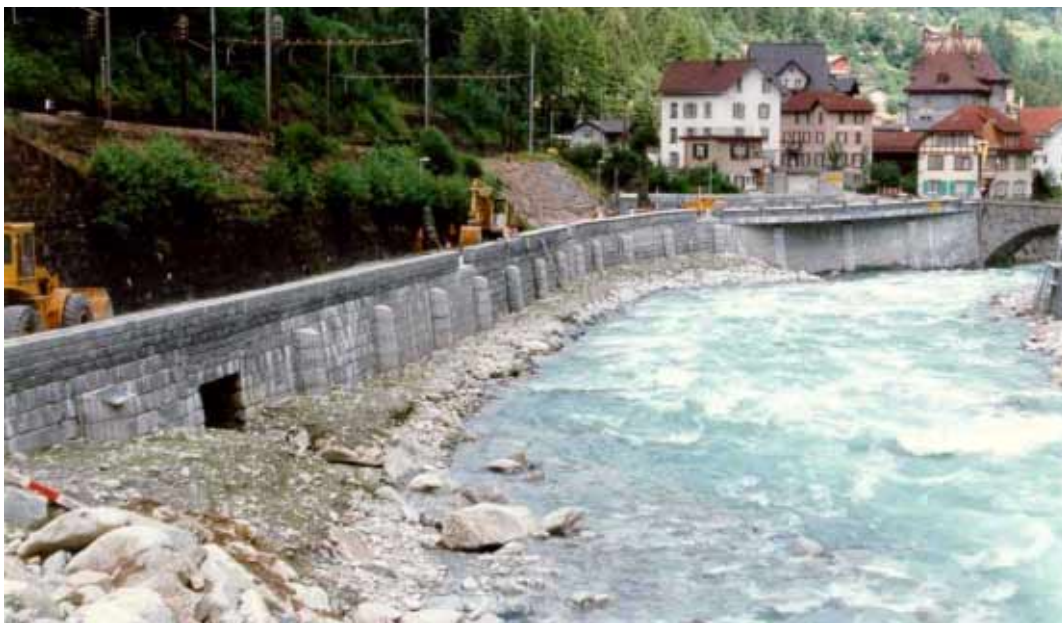
Figure 4.12: Macro-roughness on the protection wall, Reuss River in Gurtellen (Switzerland)
