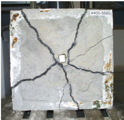
Figure 19 FRSC-slab after the puncture-flexure test.
