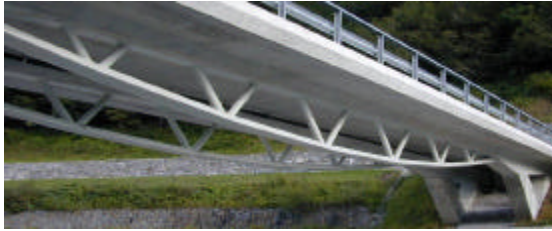
Figure 8. Tensile members for underspanned structures, possible replacement of a metallic tie by a UHPC pre-stressed member (Muttoni, 2003)
