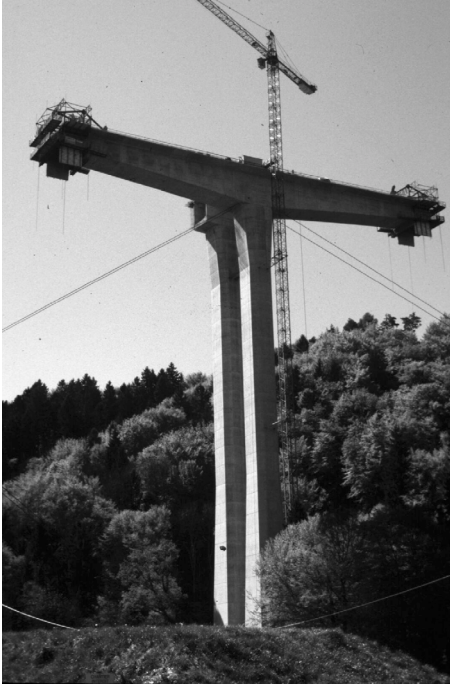
Figure 3: Pier 3 of the Mentue bridge during the free cantilevering
