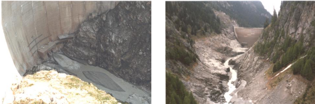
Figure 2: Flushing operation at Gebidem left) Downstream part of the bottom outlet; right) Natural transport process in the reservoir
