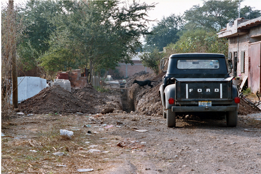
Image 34: Ongoing works to supply sanitation services in Oriente
