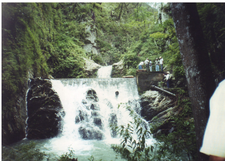
Image 21: Dam supplying the Manantlán system with pipeline
