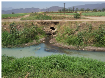
Image 27: El Grullo sewage discharge in the River
