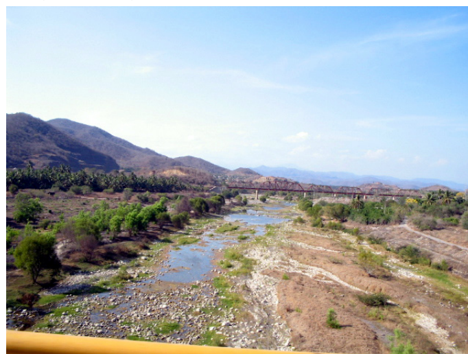
Image 45: Bridge over the Armería River in Colima
