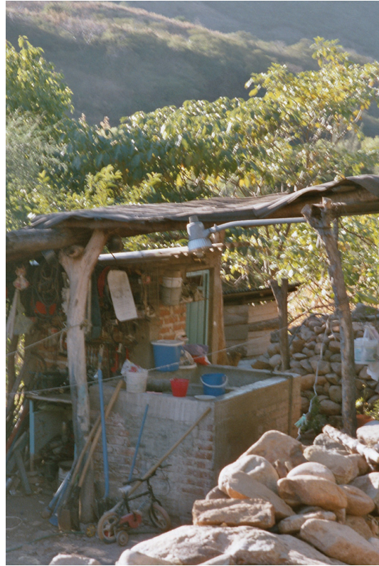
Image 39: Wash-house in La Laja
