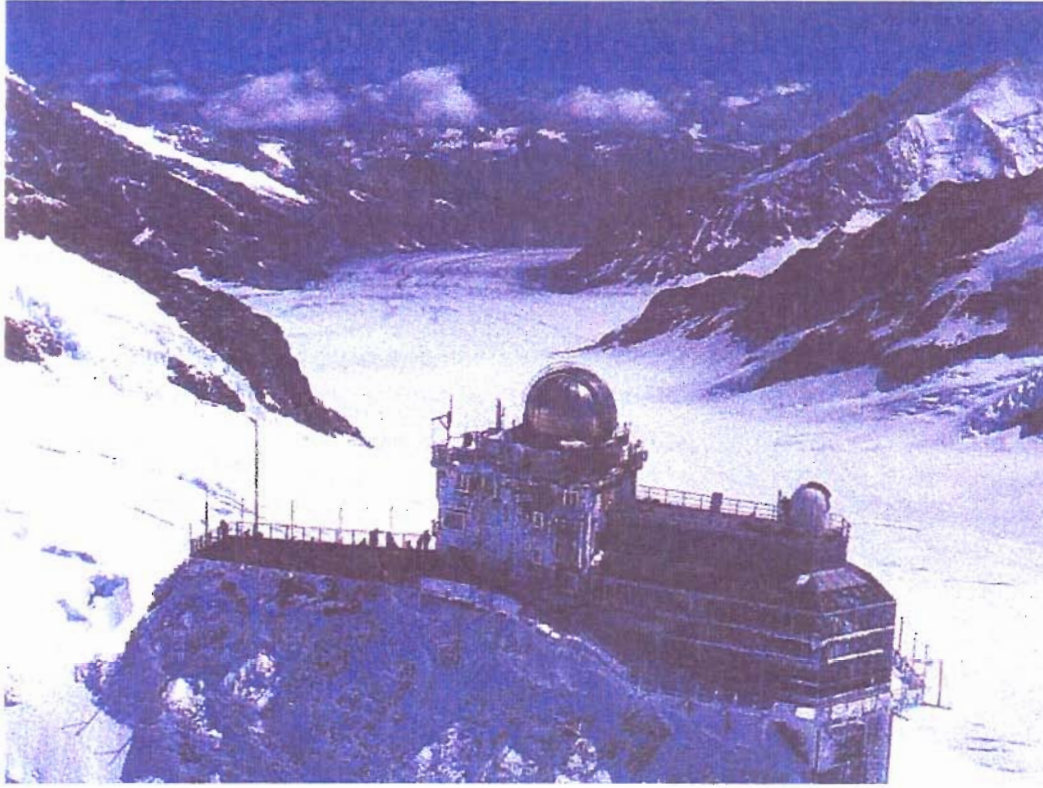
FIGURE 1. General view of the Jungfrauoch observatory and the Aletsch Glacier. The lidar system is installed inside the astronomical dome whereas the small cupola contains the sunphotometer of the Swiss Meteorological Institute.
