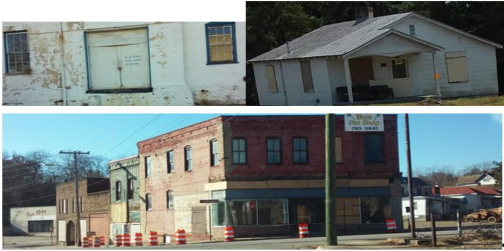
Figure 5. Blighted buildings. Photographs by A. Kautzman, 2016.
