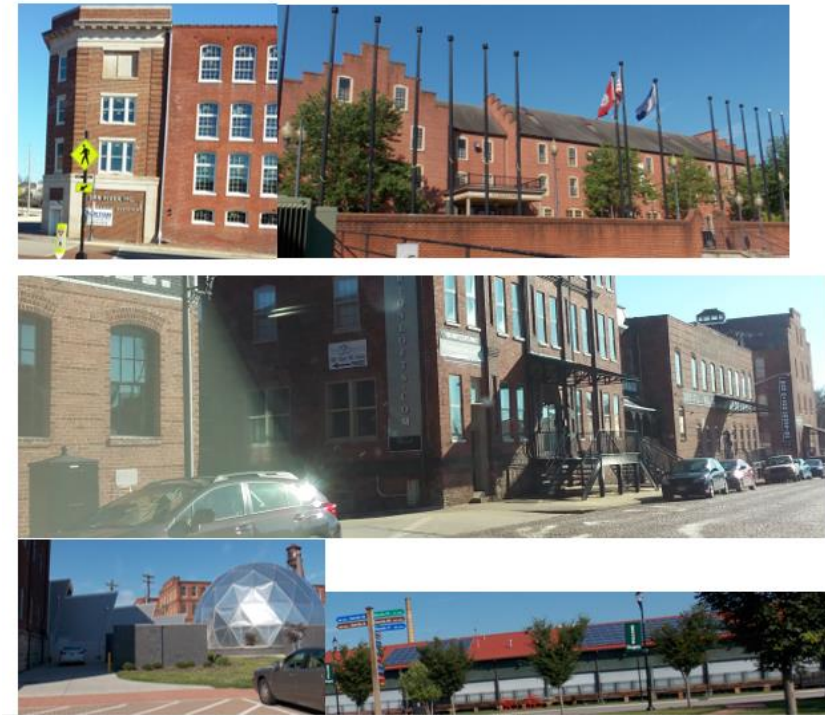
Figure 7. Bridge Street, The River District, Danville, Virginia. Photographs taken by A. Kautzman, 2016. Top left is the former Dan River R&D building undergoing rehabilitation into an orthopedic medical center. Top right is a former tobacco warehouse now occupied by the Danville Regional Foundation and Averett University’s School of Nursing. Center photos show warehouses converted to lofts and the restored cobblestone street. Bottom left is the Danville Science Center. Bottom right is the Community Market, which also serves as an event venue.
