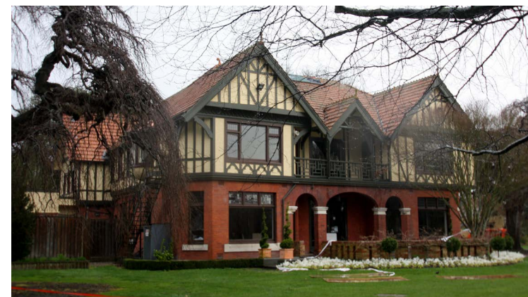
Mona Vale Christchurch Christchurch earthquake 22 February 2011, Mona Vale homestead, photograph by Ann (Helen) Devereux, Wikimedia Commons
