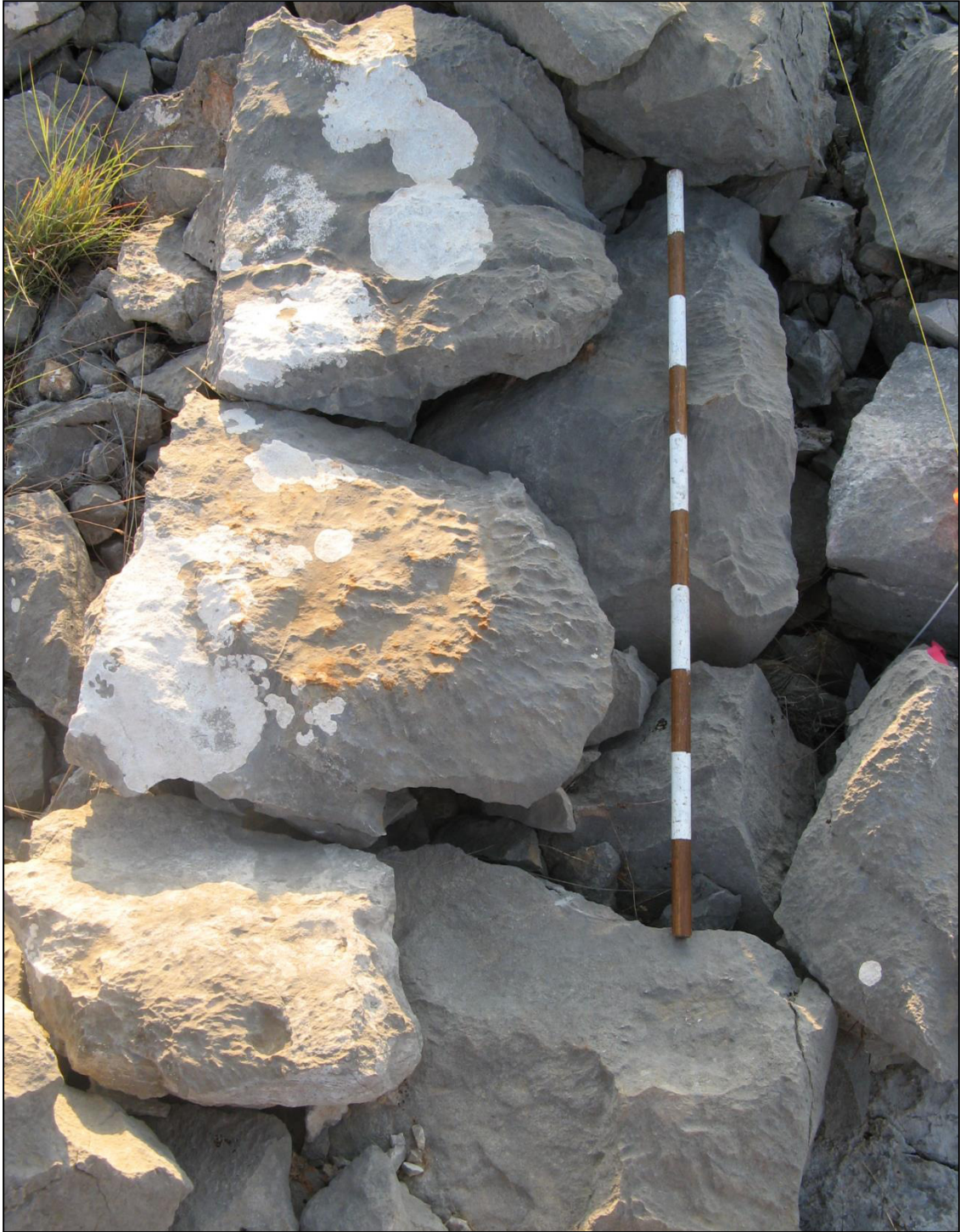
Figure A.53 Western portion of wall 408 in structure 4-VI facing east showing typical wall construction.
