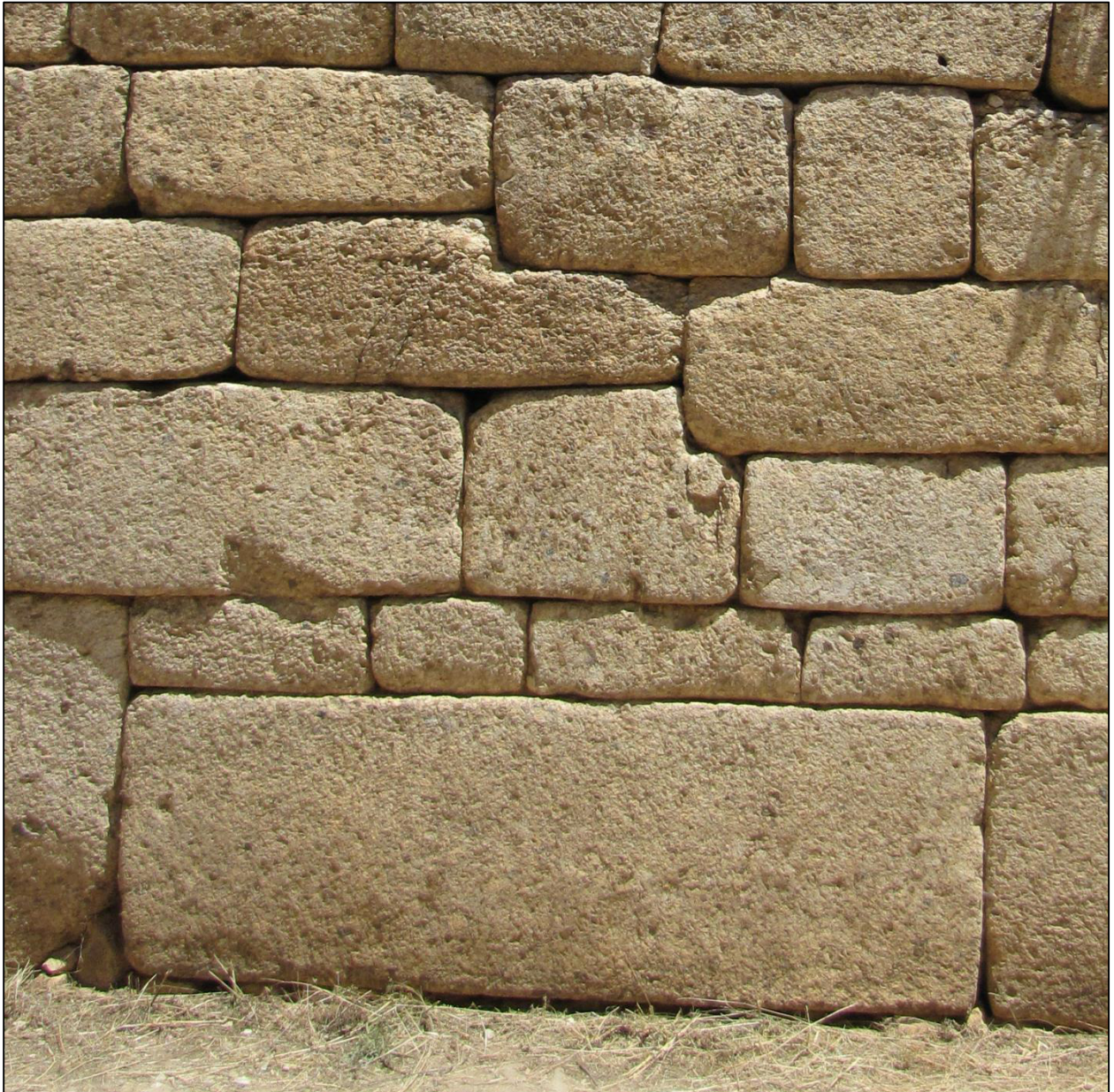
Figure A.17 The north dromos wall of the Treasury of Atreus c. 14 m from the façade showing L-shaped blocks or “hookstones” and rounding of block edges and corners.
