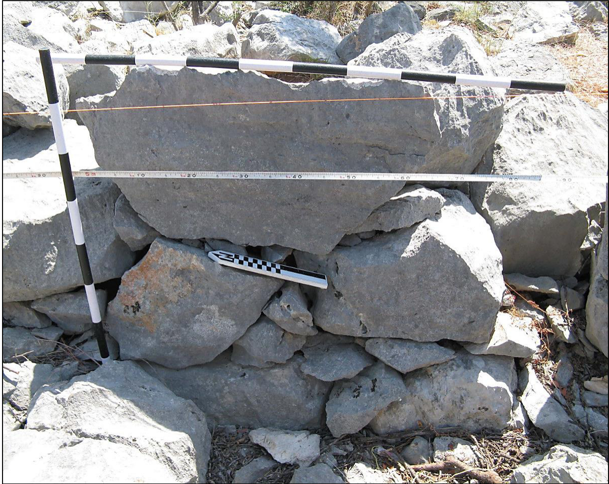
Figure A.54 Western face of wall 403 in structure 4-VI showing the use of chinking between larger, irregular stones.
