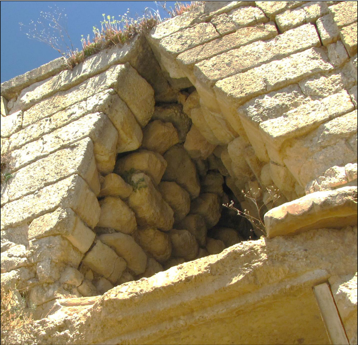
Figure A.34 A view into the Tomb of Clytemnestra's relieving triangle showing unworked conglomerate stones.
