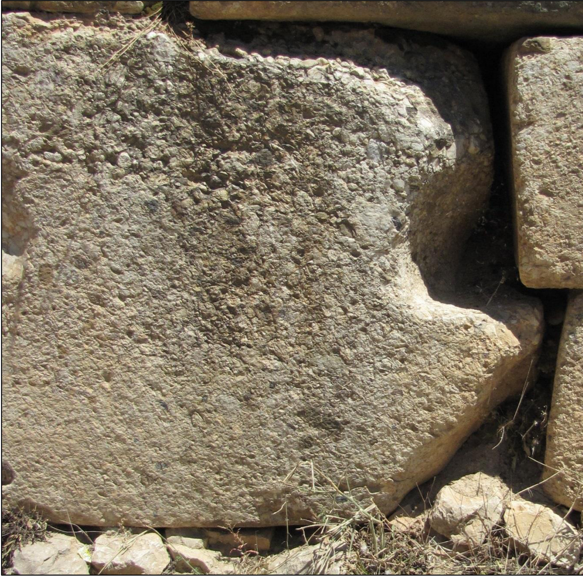
Figure A.40 Closeup of the large block in the north dromos wall of the Treasury of Atreus showing the location for a rope and lever.
