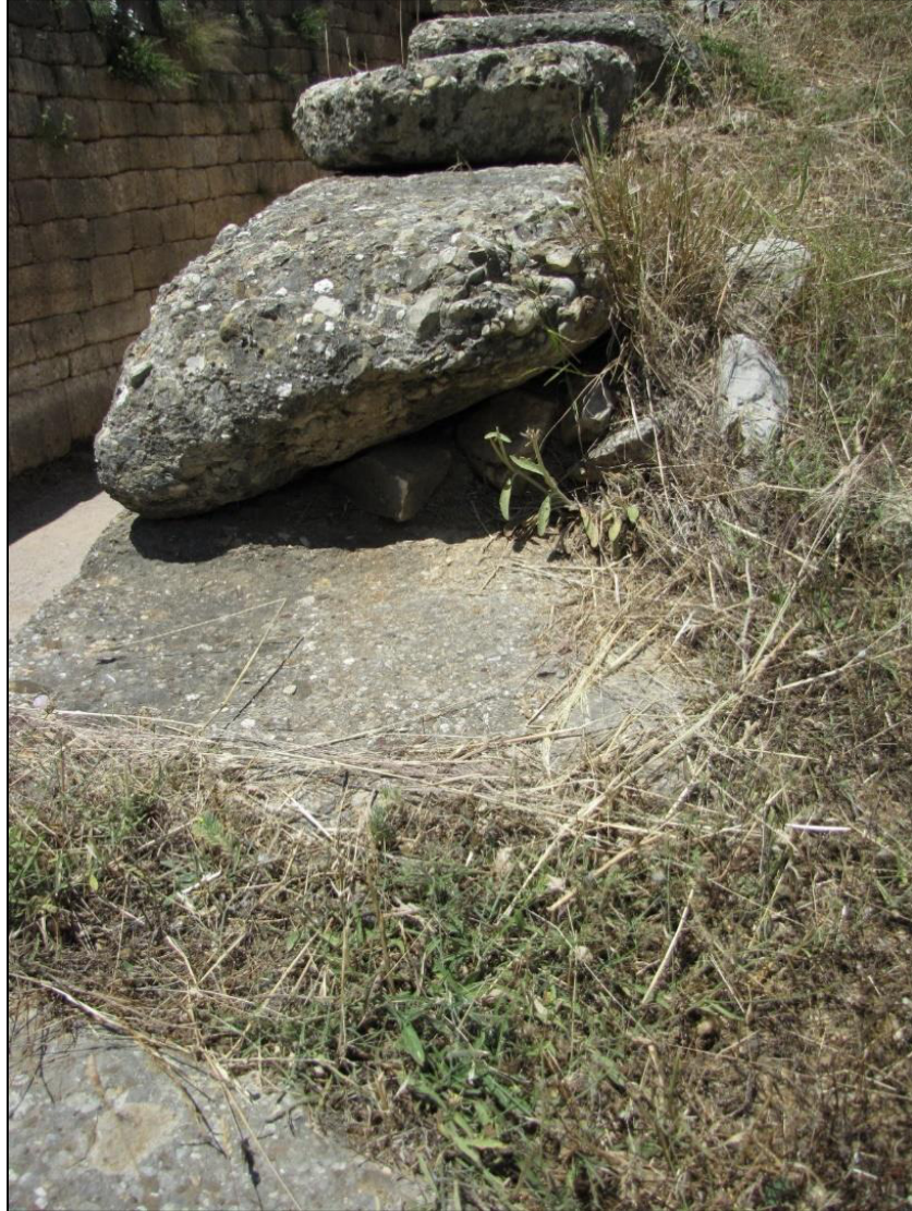
Figure A.43 A roughly dressed coping stone from the Treasury of Atreus' dromos, showing the use of chinking
