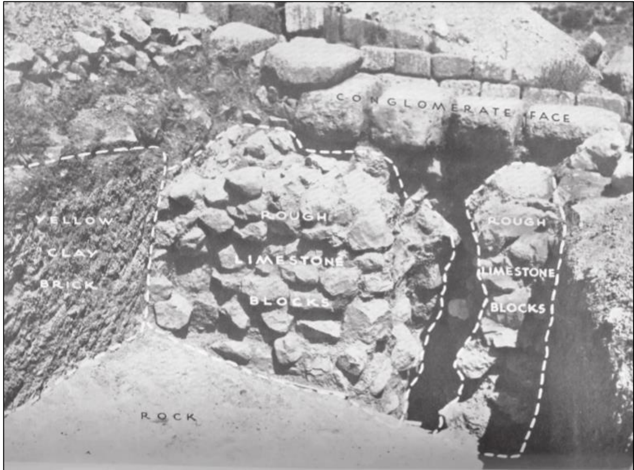
Figure A.18 Excavations behind the south dromos wall of the Treasury of Atreus showing a mortared rubble and claybrick backing (Wace 1940, pl. II).
