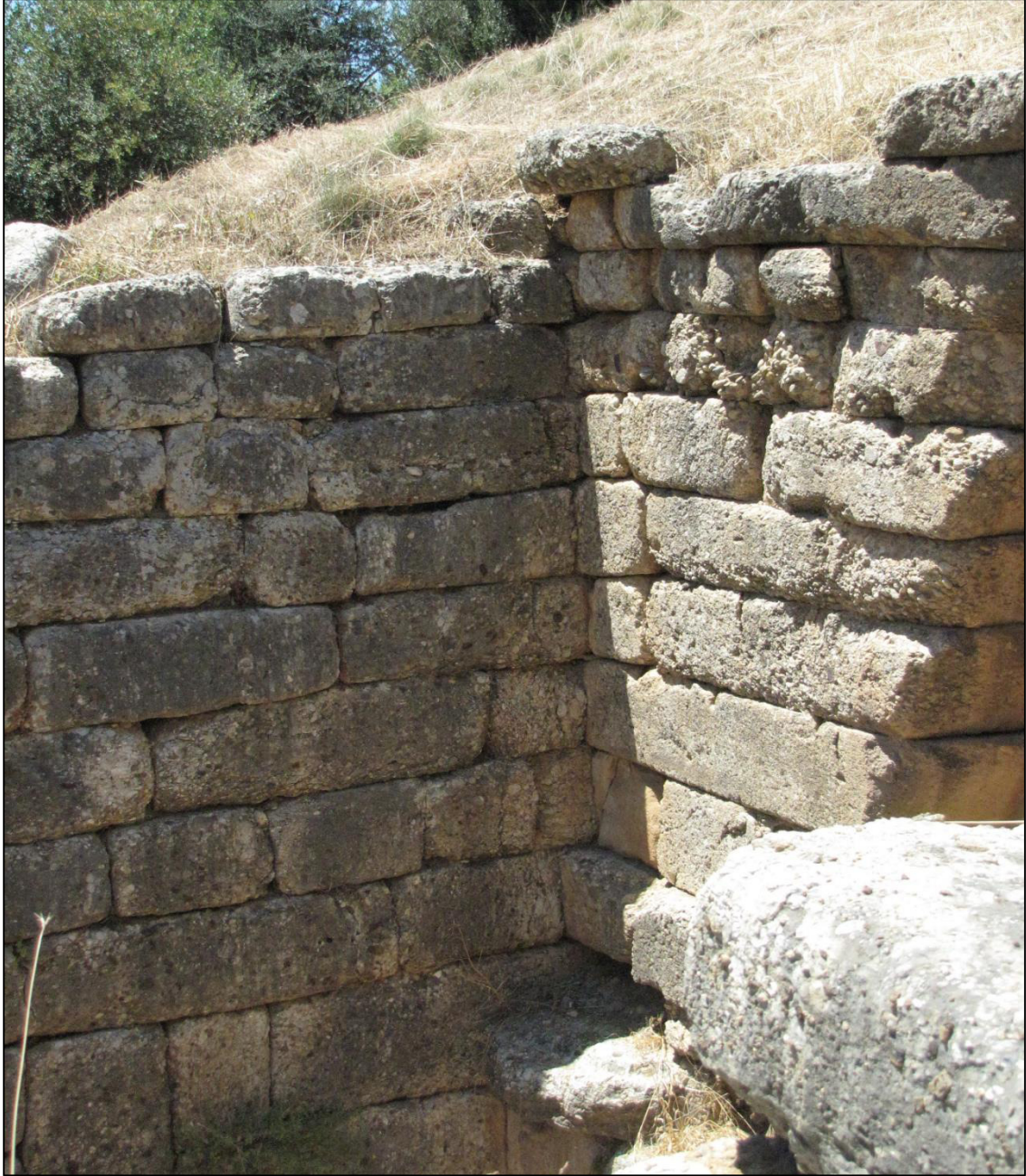
Figure A.42 The meeting of the south dromos wall and the upper façade in the Treasury of Atreus.
