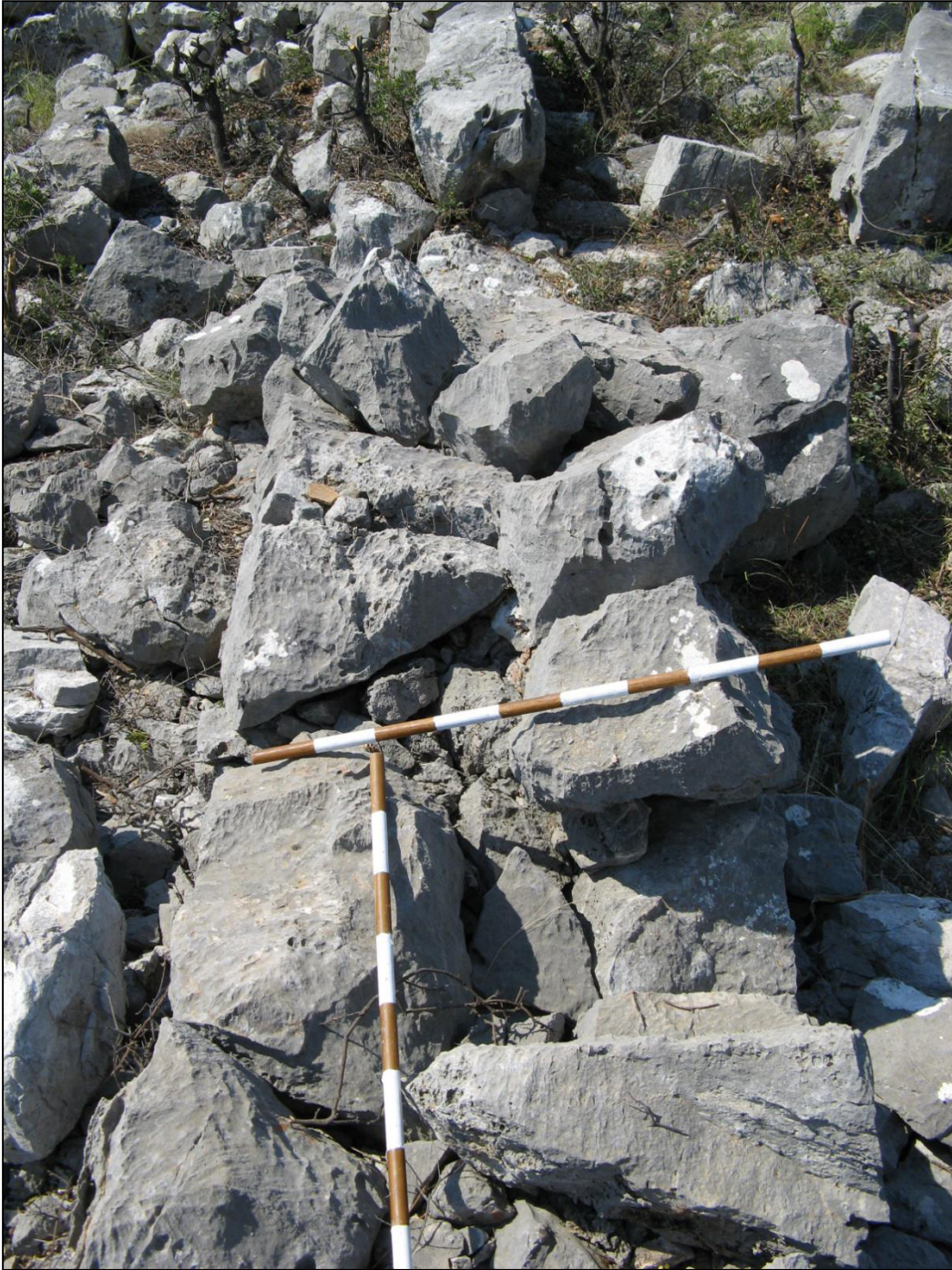
Figure A.63 Overview of wall 270 in structure 7-X facing south showing the manner of wall construction.
