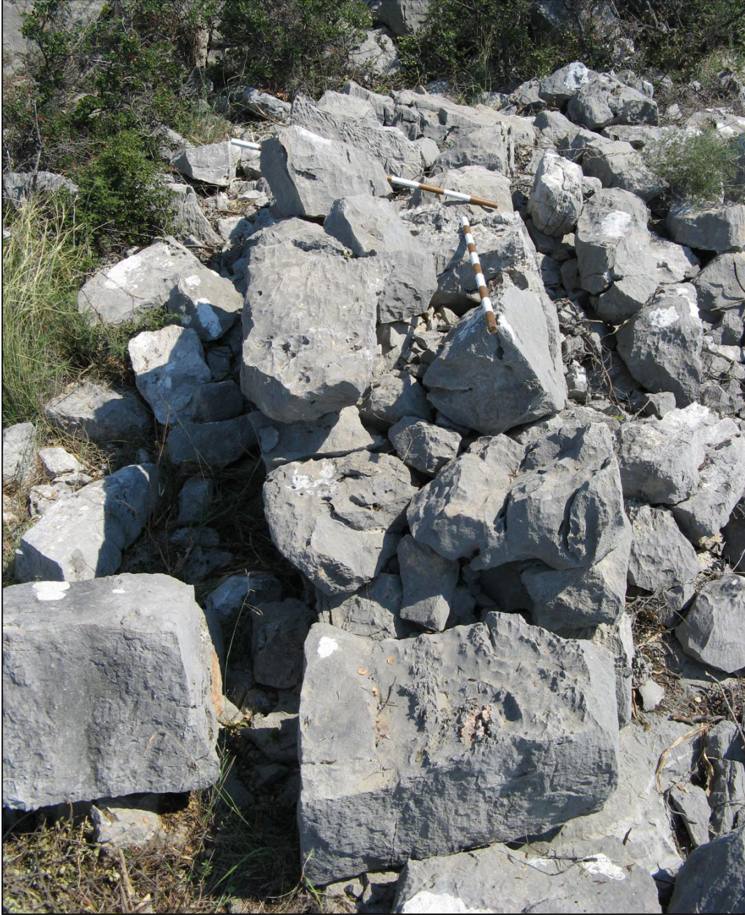
Figure A.60 The antae blocks on the north end of 7-X's main entrance.
