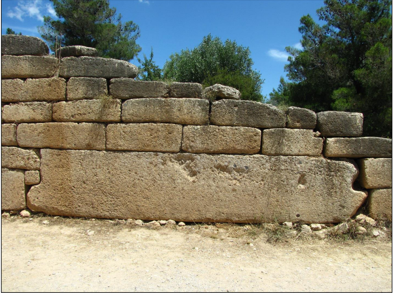
Figure A.39 The large block in the north dromos wall of the Treasury of Atreus. The block is worked to receive a rope and lever.
