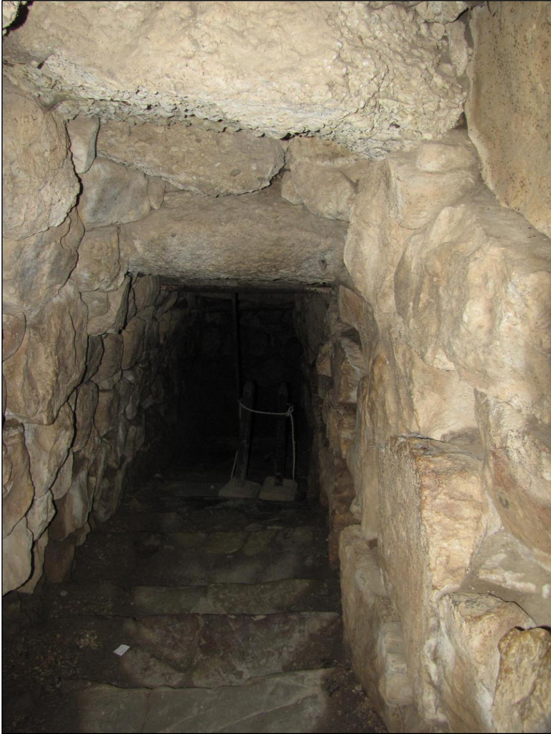
Figure A.92 The stepped passage of the underground cistern, descending to the west from the first landing.
