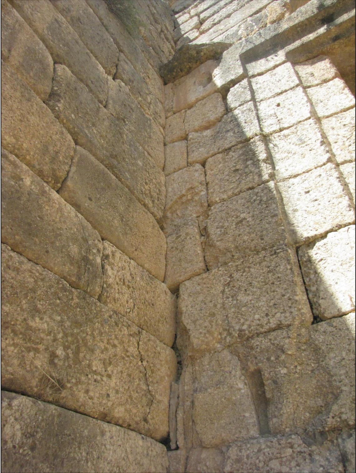
Figure A.21 The south dromos wall and façade of the Treasury of Atreus.
