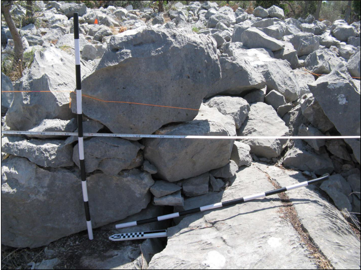
Figure A.52 Exterior face of wall 403 in structure 4-VI showing how courses were set on flattened bedrock with small leveling stones inserted.
