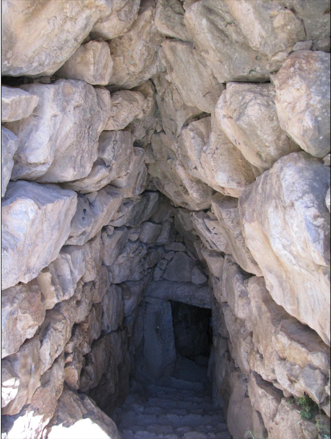
Figure A.91 The corbelled entrance to the underground cistern in the Northeast Extension.
