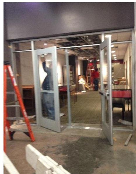
Installation of Storefront
