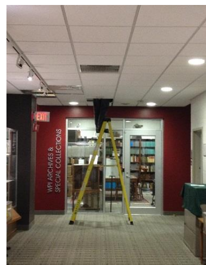
Completing hook up of new ductwork
