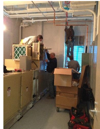
Installation of Munters HVAC unit
