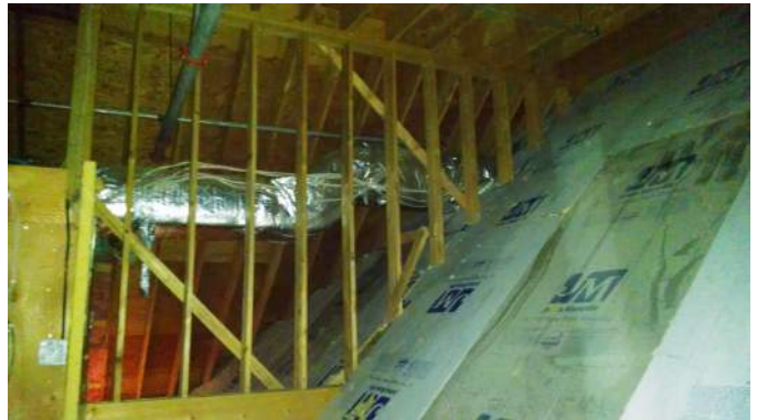
This is the attic-side of the same ductwork.
