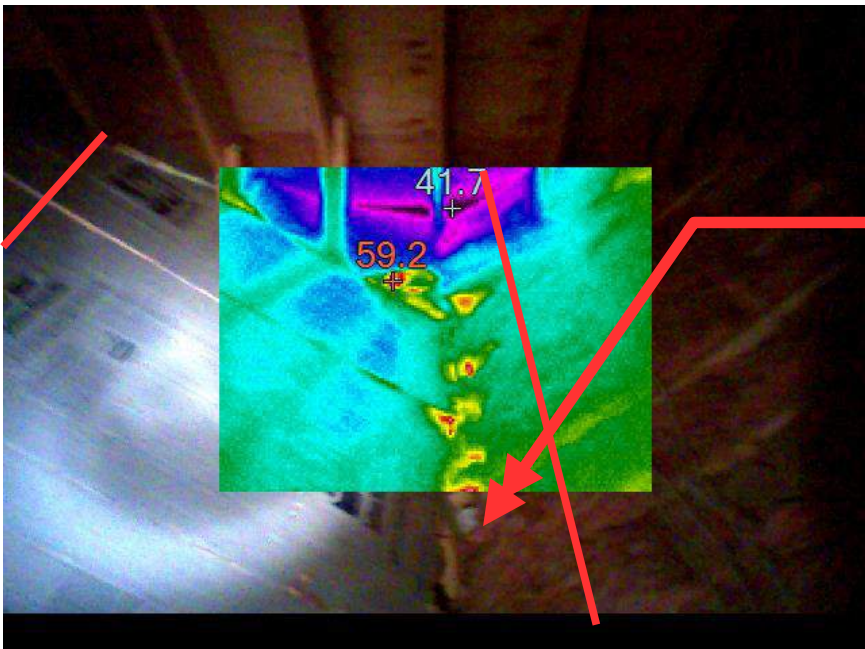
East-facing eave of exhibit room, above common-wall with hallway.
