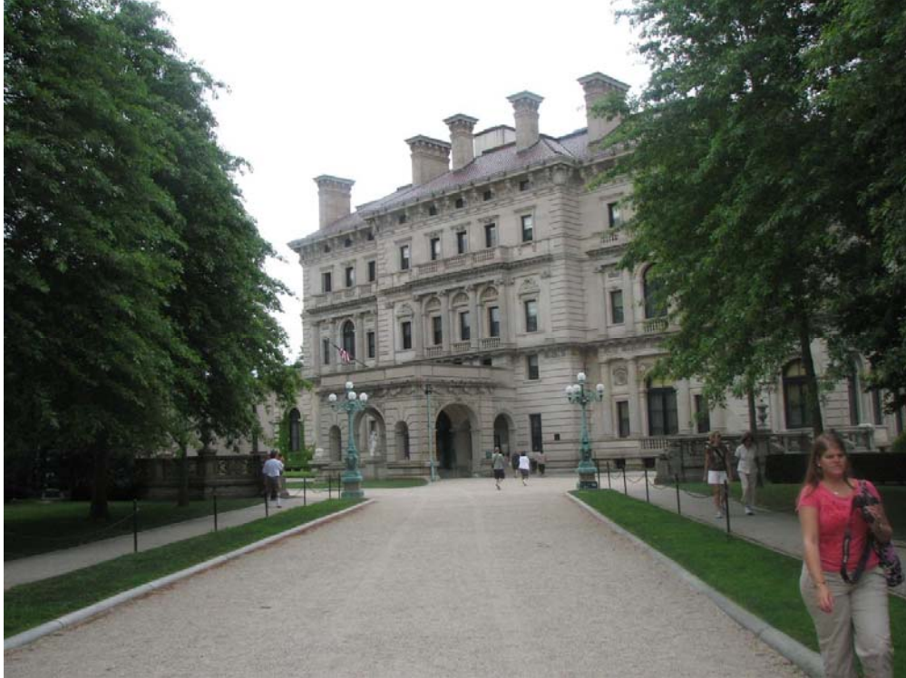
Figure 1: The Breakers, west front
