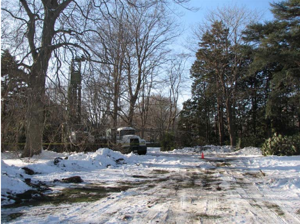
Figure 21: Drill rig path to Drill Target #2.
