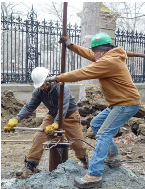
Figure 11: Adding drill rod
