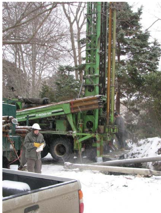
Figure 12: Drilling Target #2 in winter conditions.
