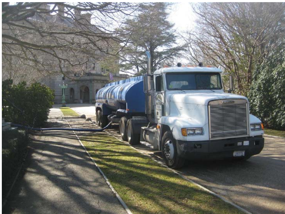
Figure 14: Water for the hydro-fracturing is supplied by a tanker truck.
