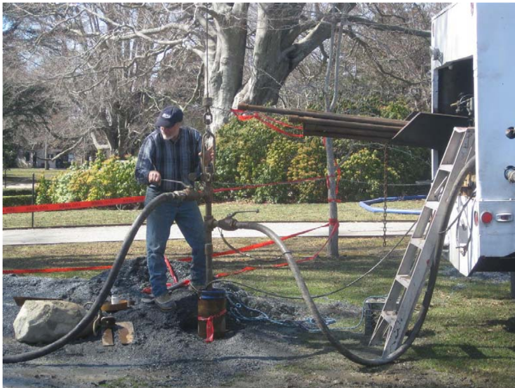
Figure 16: Well driller Joel Russell manages the hydro-fracturing operation.
