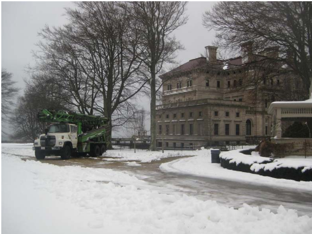
Figure 9: Drill rig arrives at The Breakers
