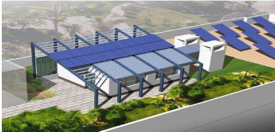
Figure 11. Solar air conditioning system installed on the rooftop of a building (Li, et al., 2007)
