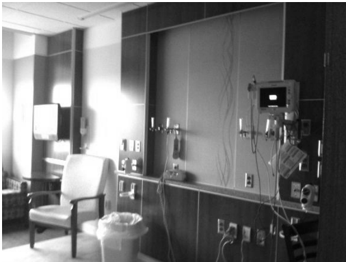
Figure 5.10: Private Patient Room Showing Head Wall
