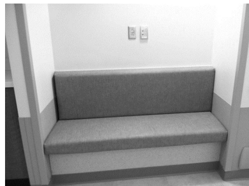
Figure 5.27: Built-in Bench in Hallway in Nursing Unit
