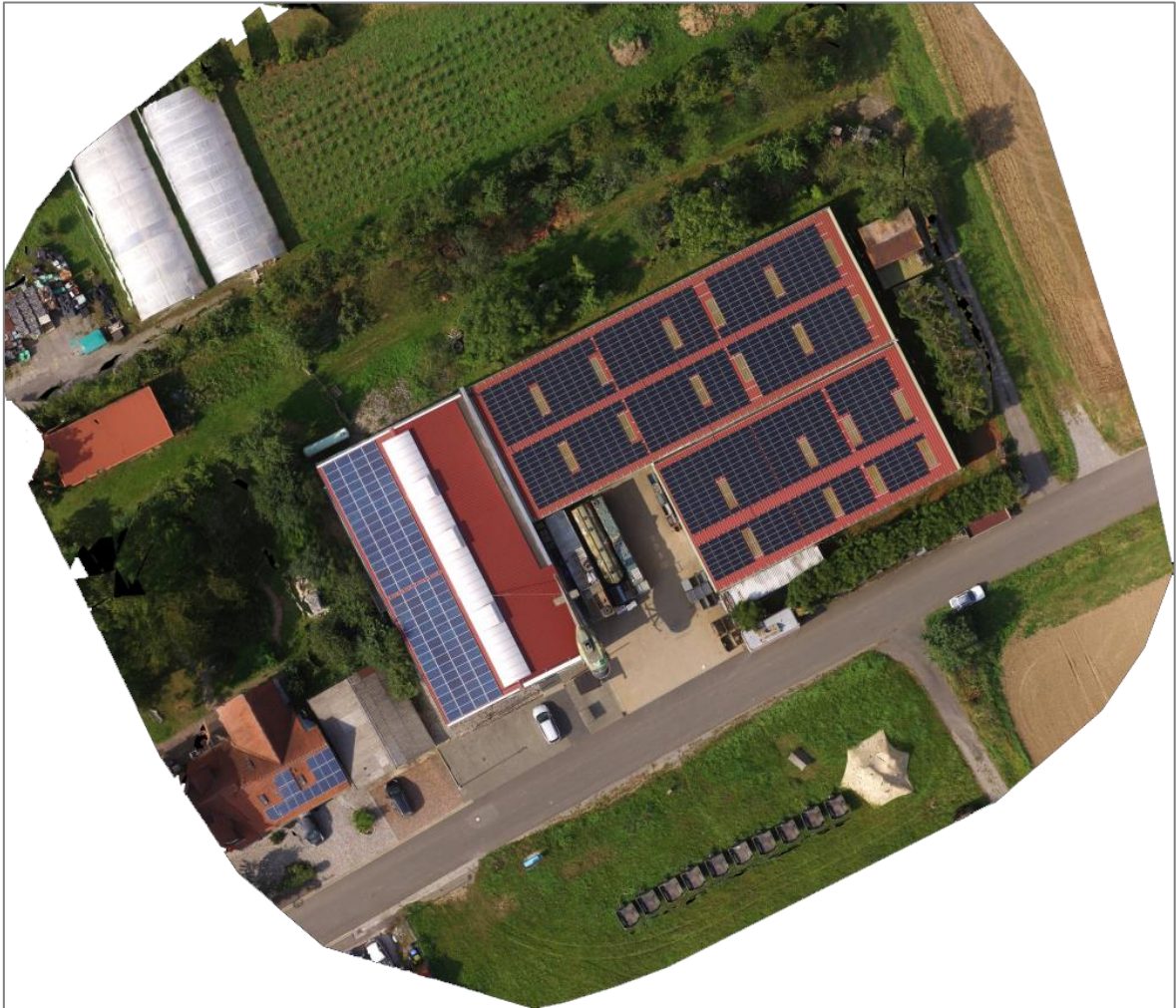
Figure 55: Orthomosaic of the PV installation at the study region
