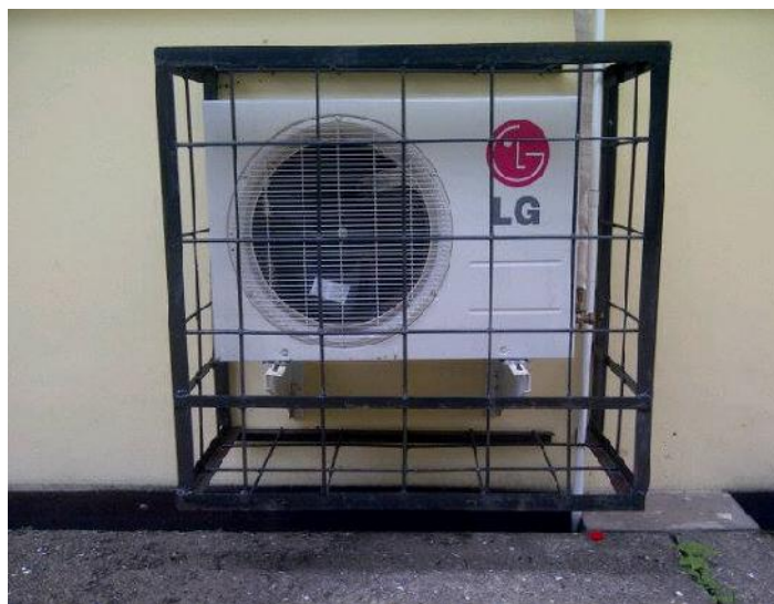
Gambar 4.1 AC Outdoor LG S18LFG 2 PK
