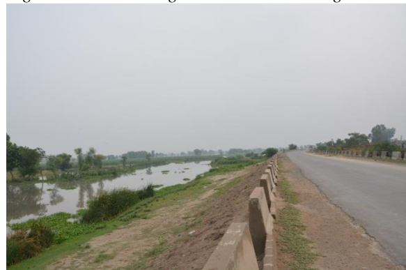
Figure 46: Untreated waste water along flood dyke
