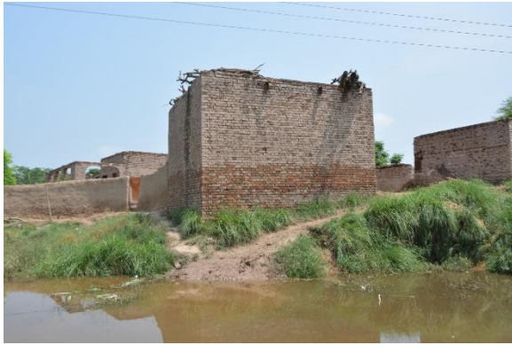
Figure 49: Raised platform of house
