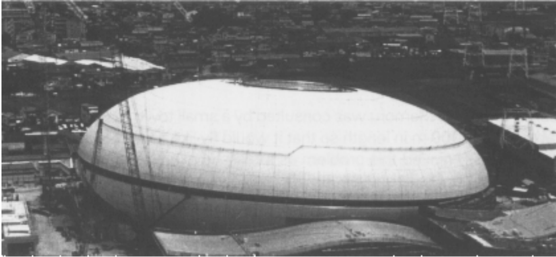
9. Namihaya Sports hall: Space frame of Pantadome System, lifted in non-vertical direction in 8,5 hours; with Showa Sekkei.
