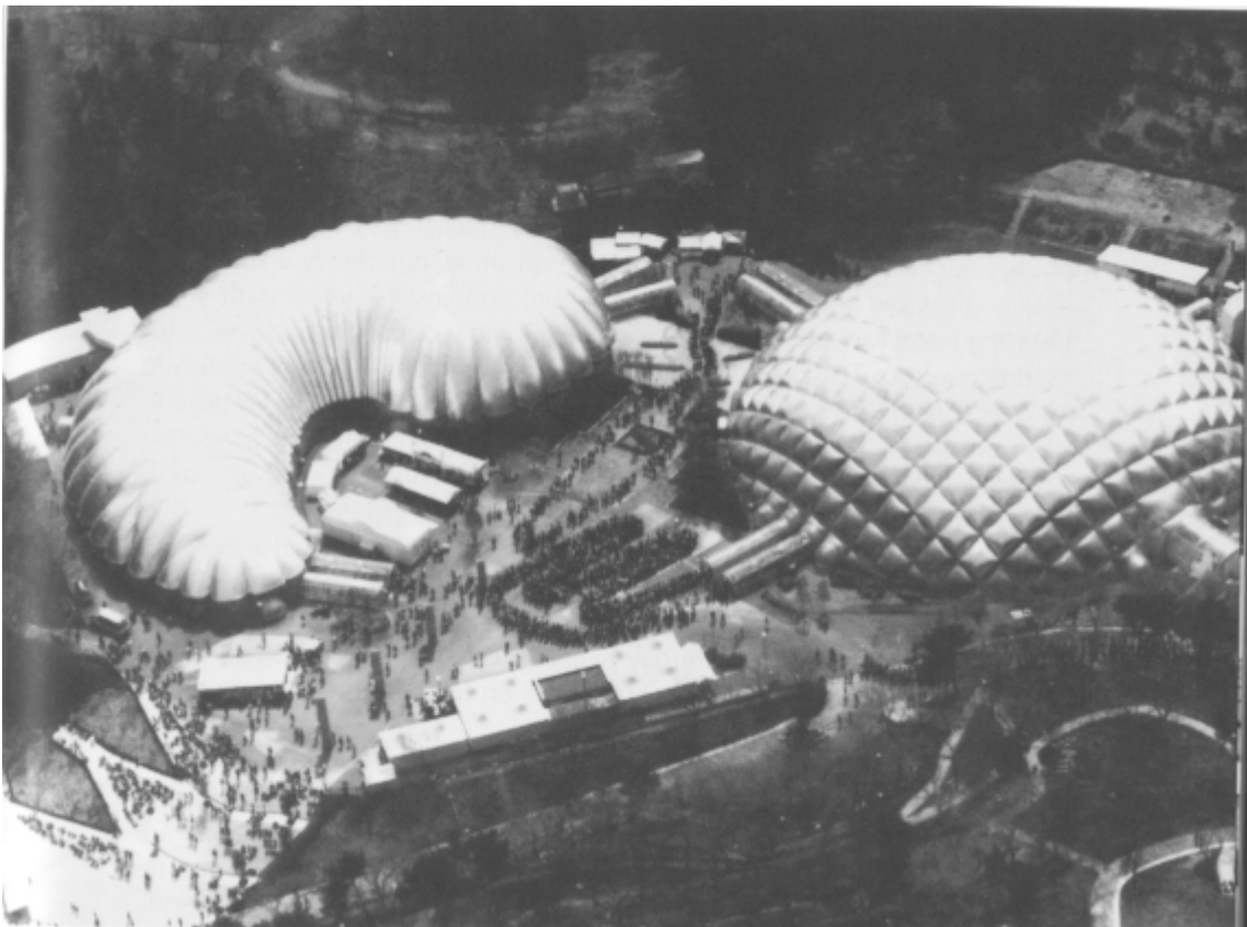
4. Pavilions for the World Conference on Orchid, Tokyo: Transparent pneumatic envelopes; with architect Y.Murata.
