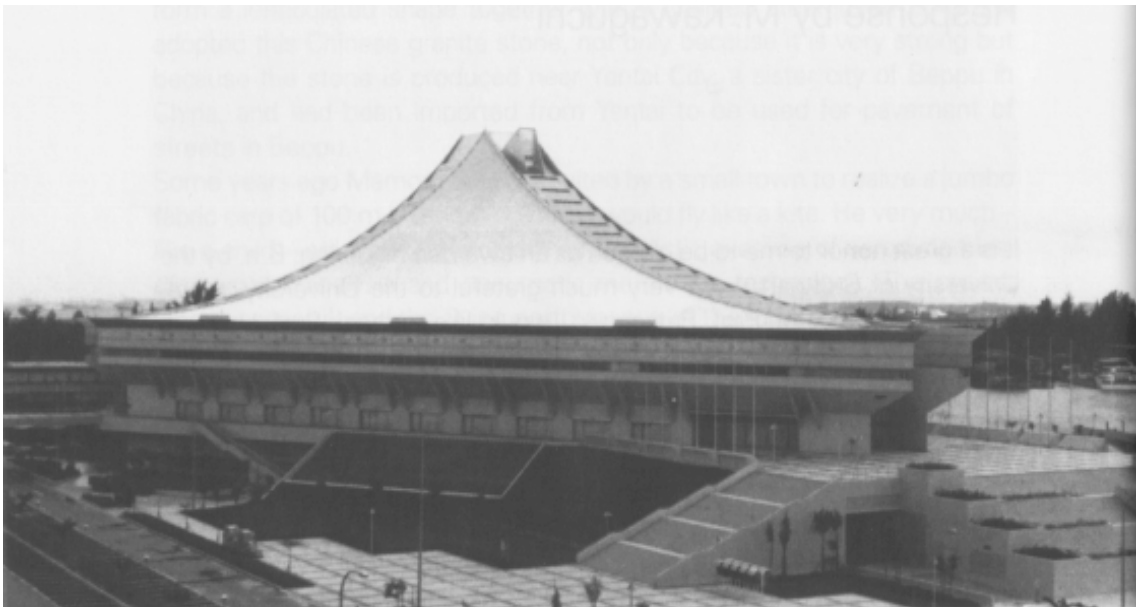
10. Singapore Indoor Stadium: Pantadome System; with K. Tange.
