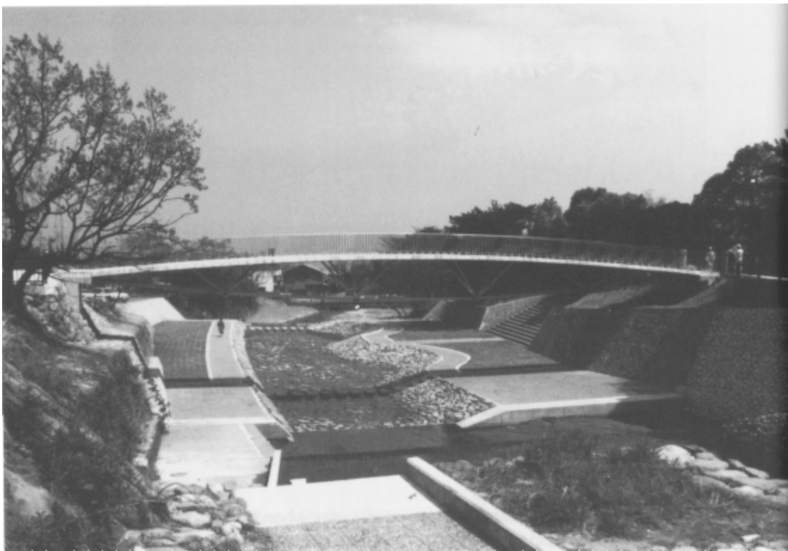
12. Inachus Bridge: Pedestrian bridge of natural granite stone; Kawaguchi played the role of architect, too.
