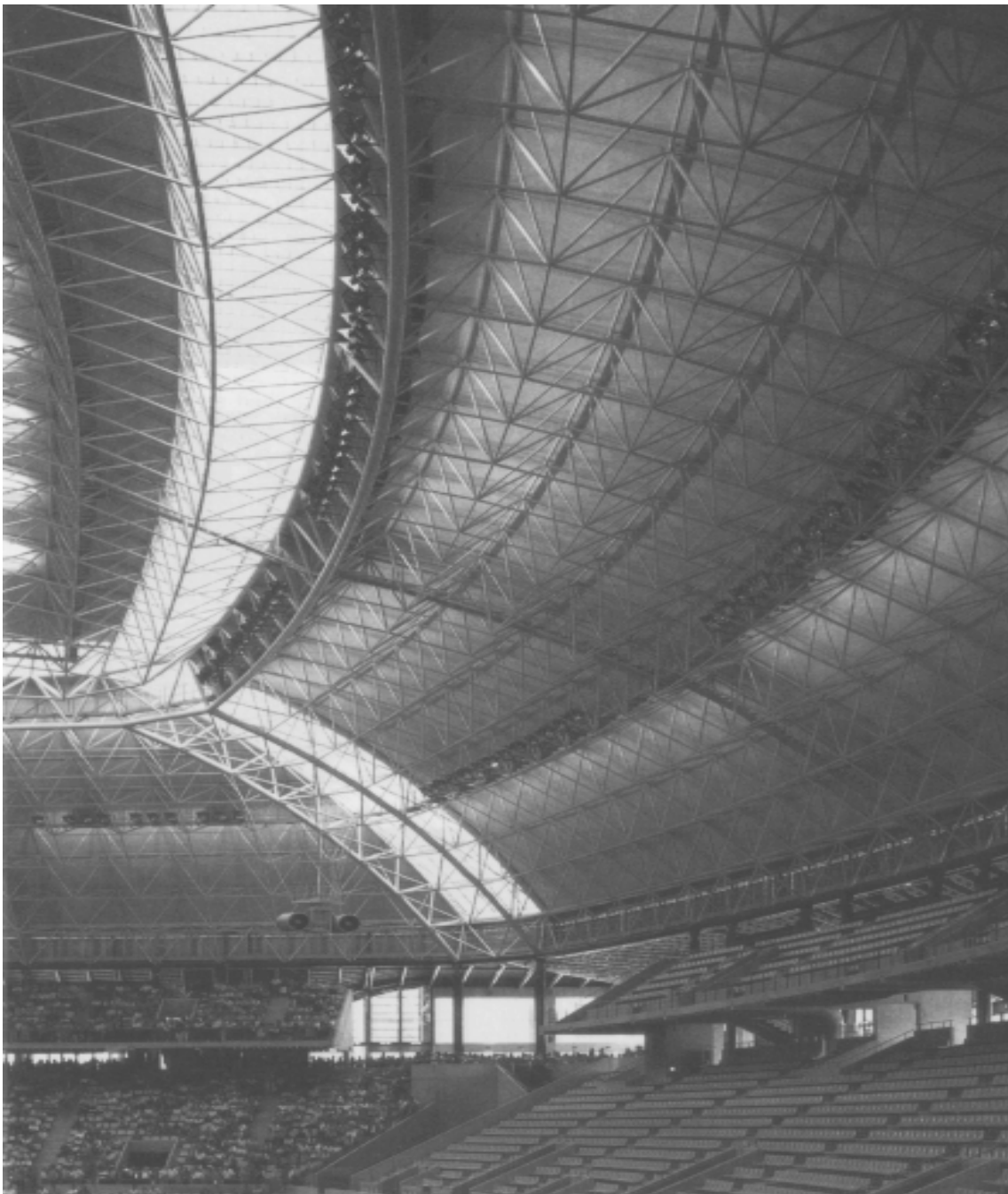
8. Sant Jordi Sports Palace for Barcelona Olympics (interior): Another Example of Pantadome System; with Architect A Isozaki
