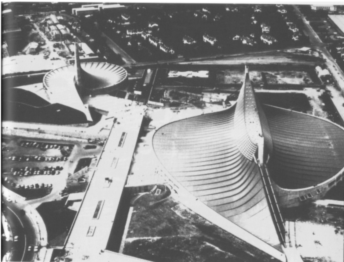
1. Yoyogi Indoor Stadium: suspension roofs by Tsuboi & Tange, the first major structure in which Mamoru Kawaguchi was involved.
