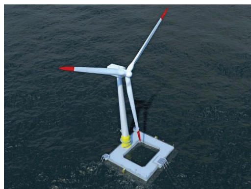
Fig. 1: Illustration of the two MW floating offshore wind turbine system within EU-FP7 project FLOATGEN (source: IDEOL)
