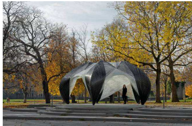
Fig. 1. First architecture built entirely by a robotic winding technique
