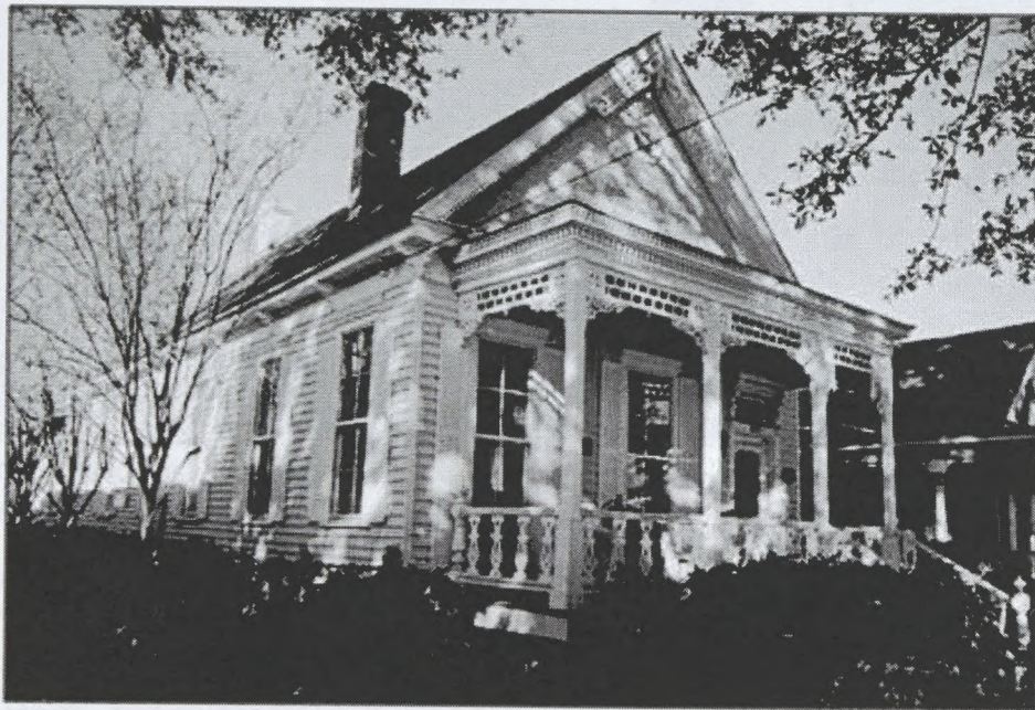
445 Broad Street appears today much as it did historically. Photo by author, 2007.
