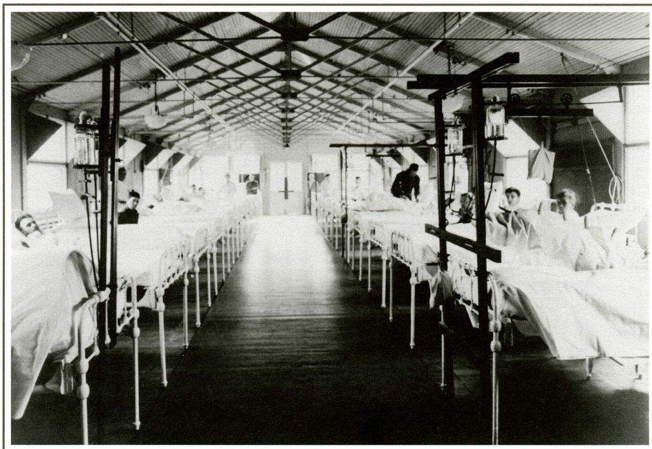
A ward in one of the temporary War Demonstration Hospital buildings.
