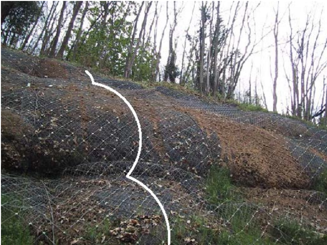
Fig. 1. Section of membrane panel represented in simulation
