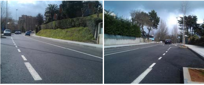
Figure 15. Road in use
