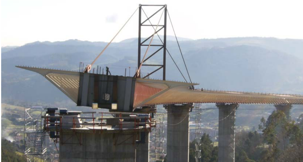
Fig. 18. Fifth launching stage of the Regueirón Viaduct.
