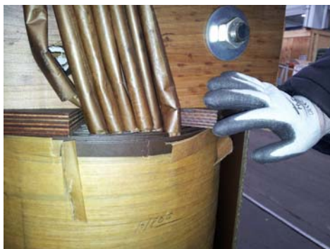
Fig. 3. Transformer studied: Detail of the inner and outer paper layers.
