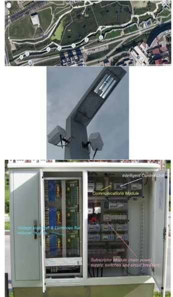
Fig. 2. Details of the field trial deployment
