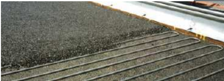
Figure 54: Geothermal snow melting and de-icing is based on hydraulic systems, European Geothermal Energy Council (2007)
