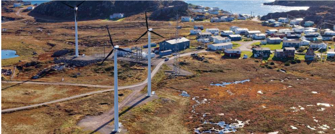
Figure 209: NL Ramea Island wind-diesel hybrid micro-grid ( http://news.cision.com )
