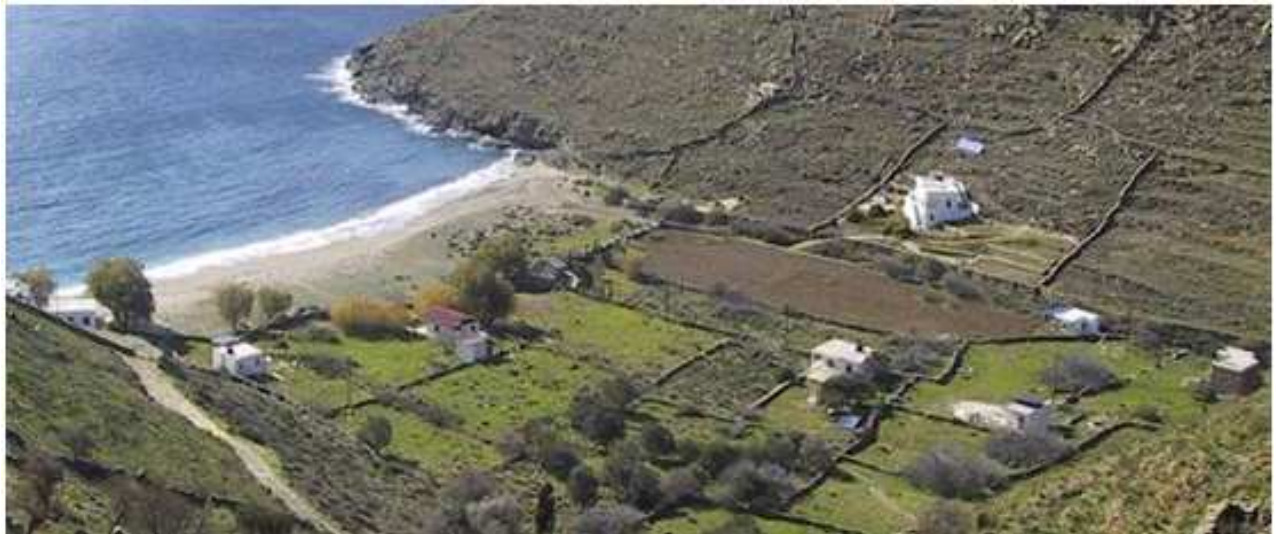
Figure 207: Gaidouromandra Microgrid in Kythnos Island: general view ( http://www.microgrids.eu/ )
