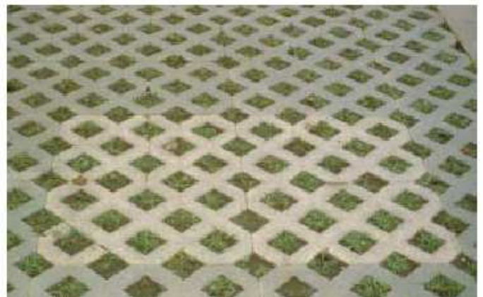
Figure 77: Concrete grids (The University of Rhode Island, 2005)
