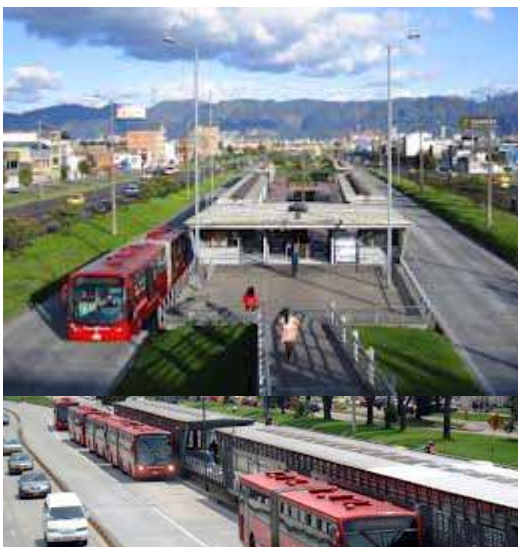
Figure 182: BRT “Transmilenio” in Colombia (Wikipedia, 2013)
