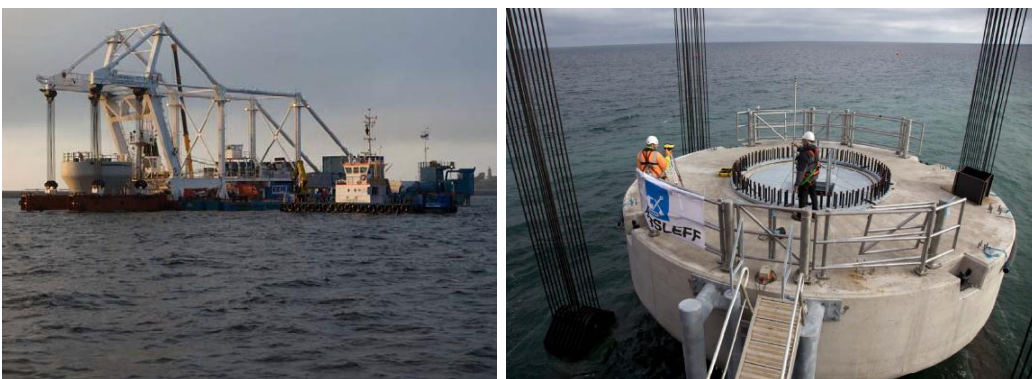
Foundation installation (ABJV)
