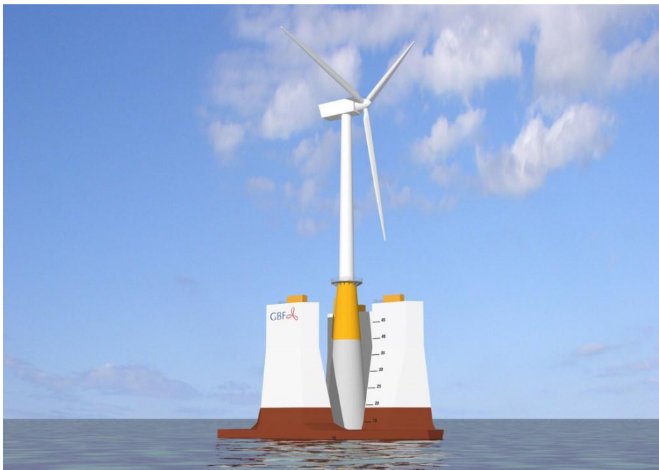
Figure 44: Complete pre-assembled turbine installation (GBF, 2012)
