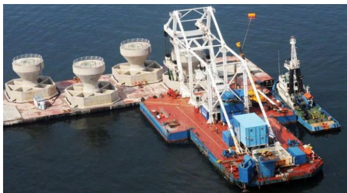
Foundations transport (ABJV)
