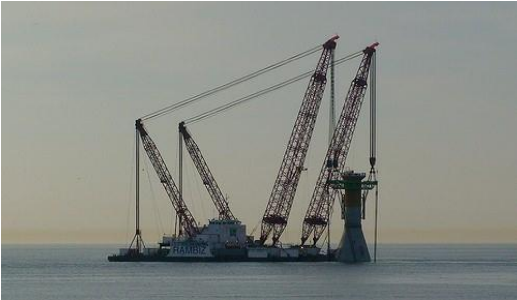
Figure 6: Foundation transport in Thorntonbank (Luc van Braekel, 2008)
