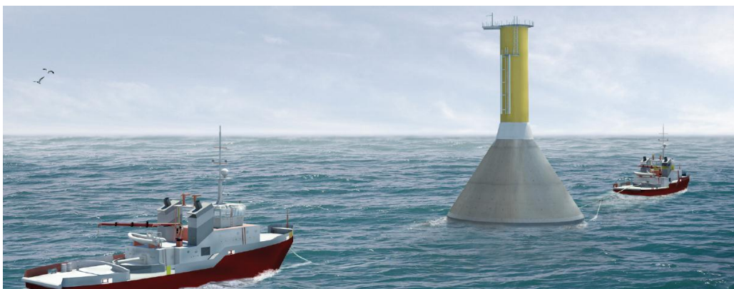
Foundation transport (Gravitas)
