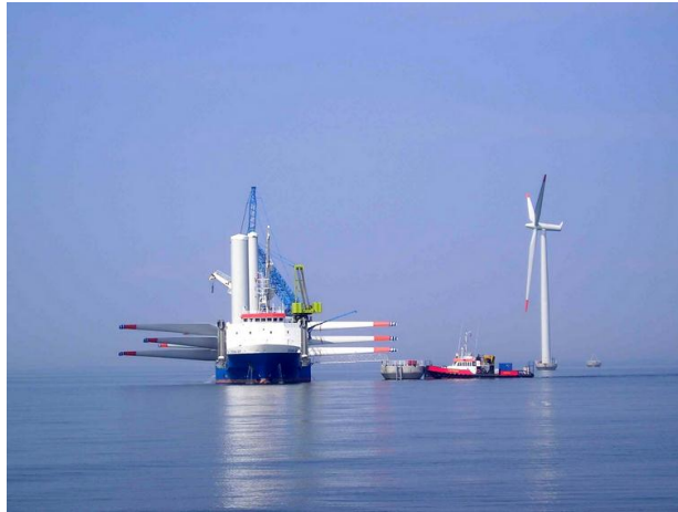
Turbine installation (EON)
