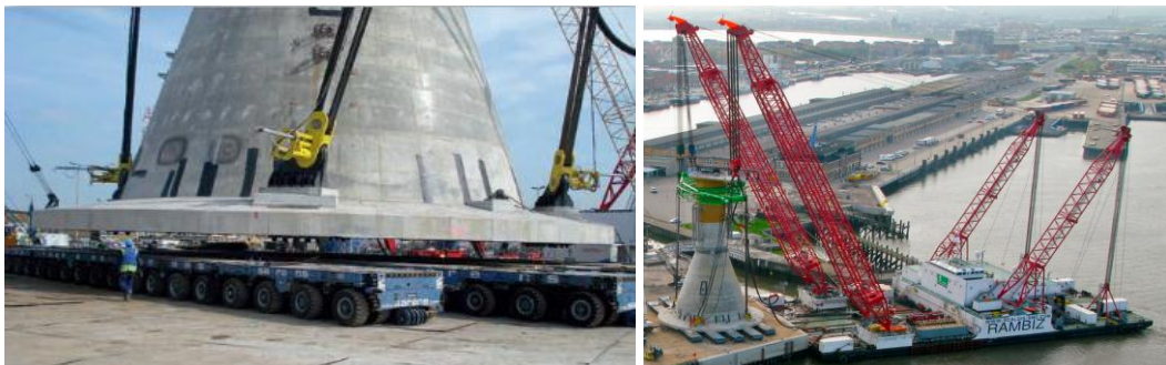
Foundation transport (left: DEME, right: Scaldis)
