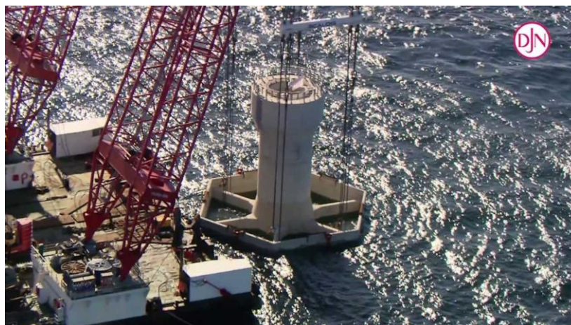
Foundation installation (Jan de Nul)
