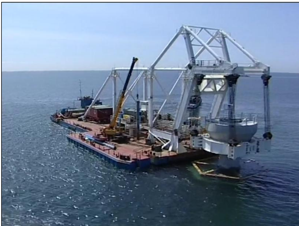
Lowering a foundation (DONG Energy)
