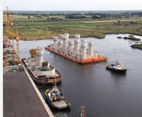
Foundations transport (Maritime journal)
