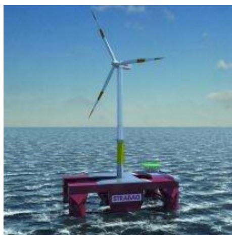
Foundation transport (Strabag)
