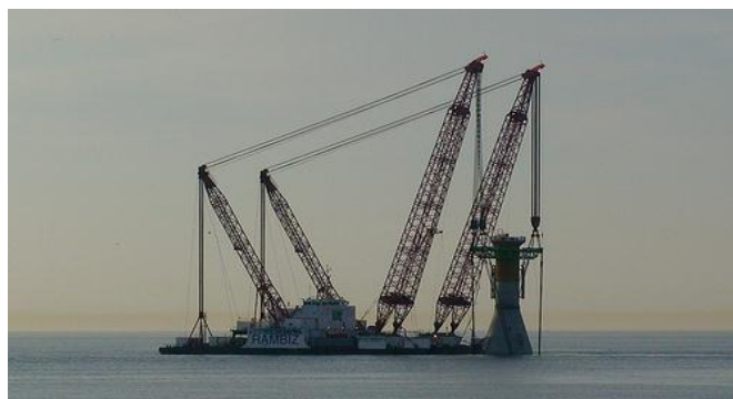
Foundation transport (IMC)
