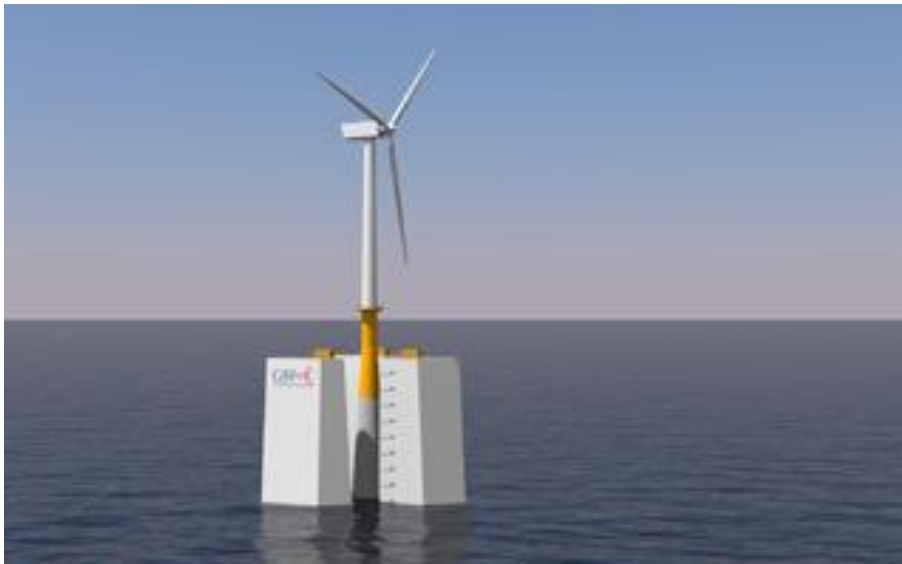
Foundation installation (GBF)
