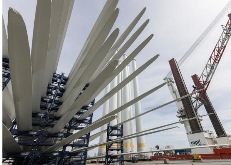
Turbine installation (renews)
