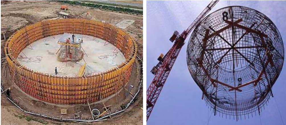
Foundation manufacture (Power technology)
