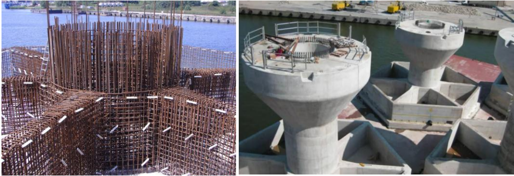
Left: Steel frames (Niras). Right: foundation Construction (ABJV)
