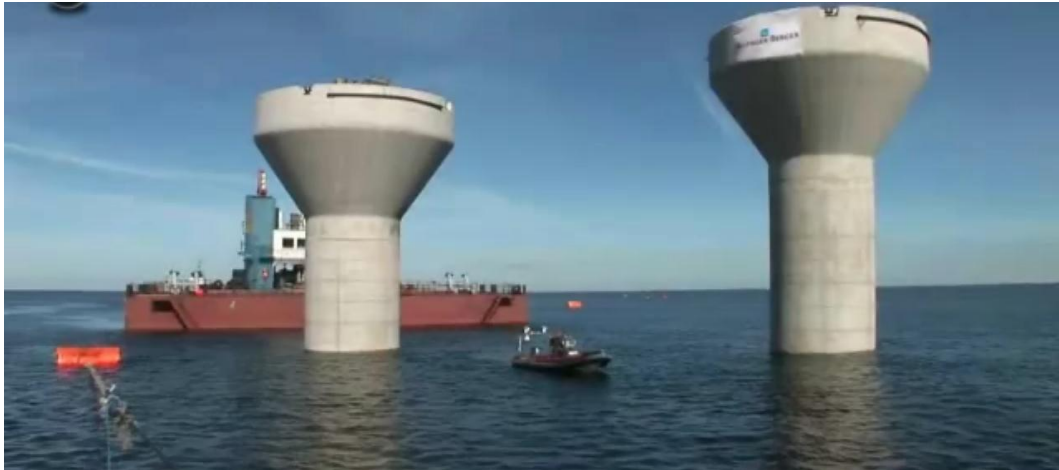
Figure 25: Pontoon partially submerged in Rødsand (ABJV, 2012)
