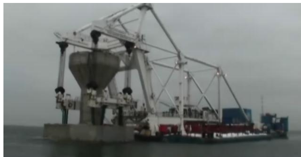
Foundation lowering down (ABJV)
