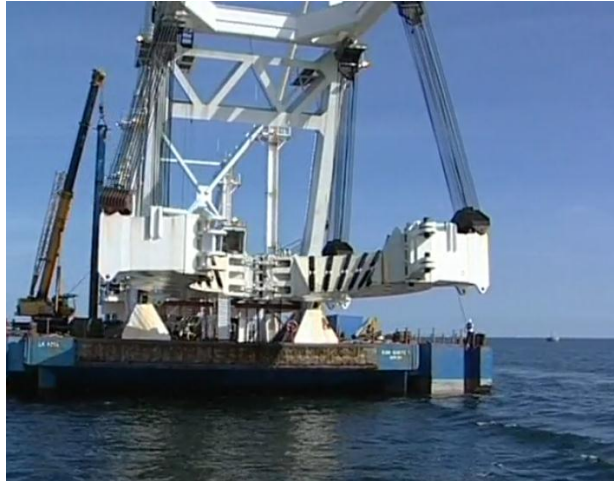
Crane Eide Barge 5 (DONG Energy)
