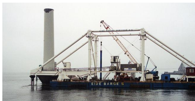
Foundation transport (Power technology)
