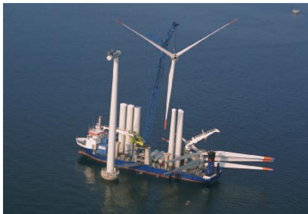
Rotor installation (DONG Energy)
