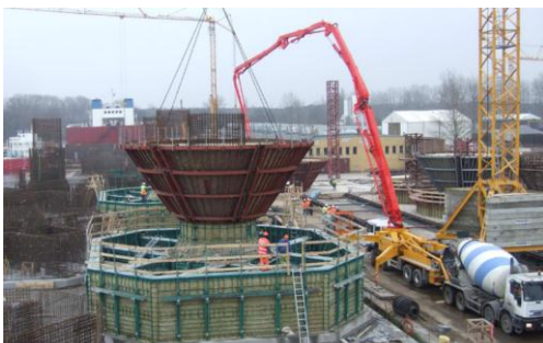
Concrete casting on barge (ABJV)
