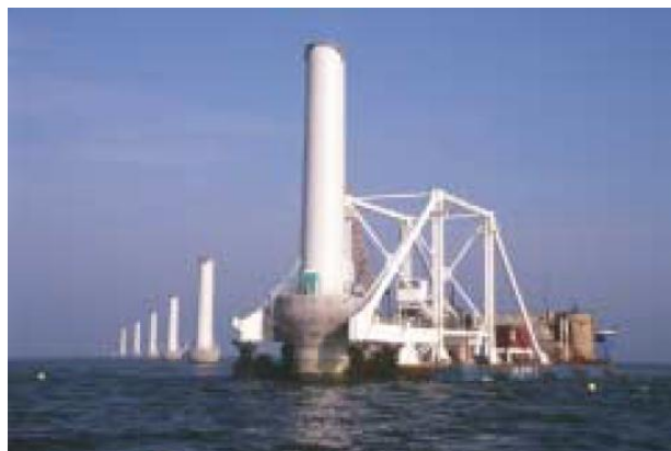
Foundation installation (ABJV)
