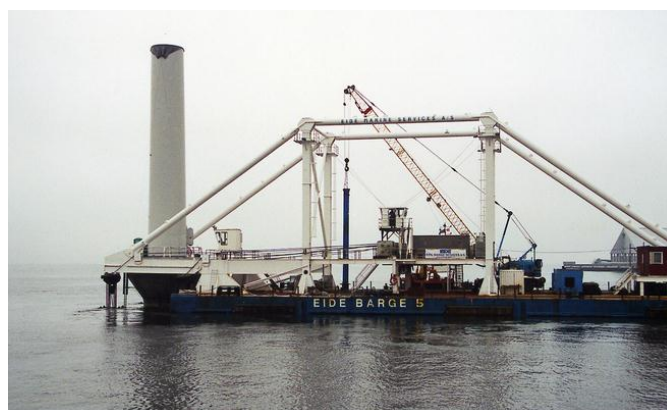
Figure 43: Foundation installation in Middelgrunden (Power technology, 2001)
