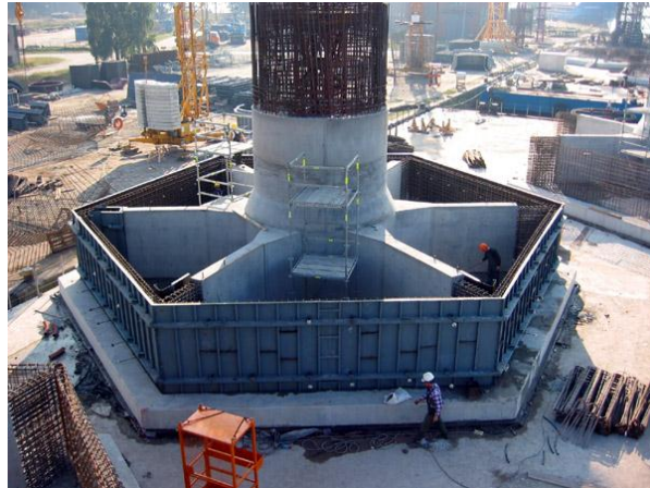
Foundations manufacture (Dong Energy)
