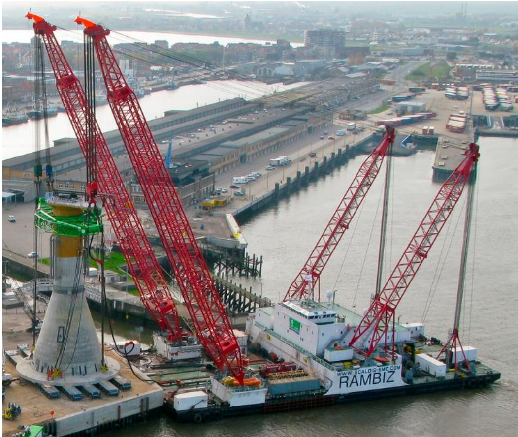
Figure 7: Foundation launching in Thorntonbank (Scaldis, 2008)
