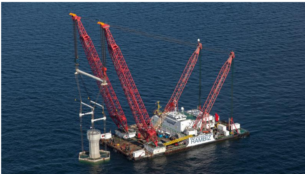
Figure 26: Foundation transport and installation by RAMBIZ (Scaldis, 2012)
