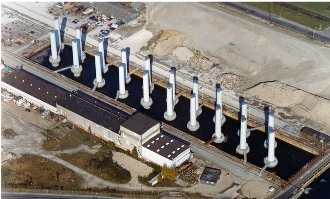
Figure 8: Foundation construction in dry docks (Aarsleff, 2001)
