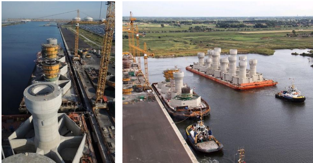
Figure 5: Foundations construction and transport in Kårehamn (Jan de Nul S/A, 2012)
