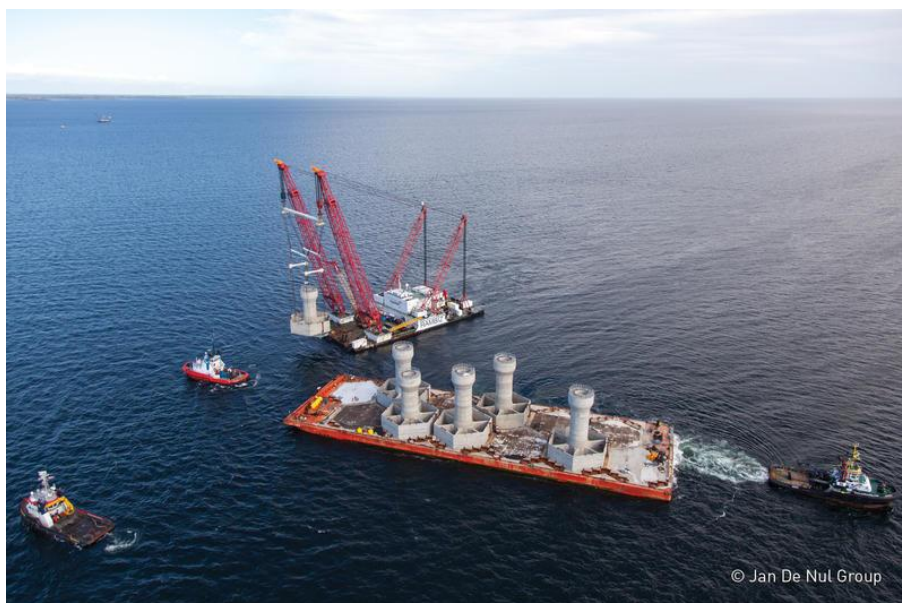
Foundation transport (Jan de Nul)
