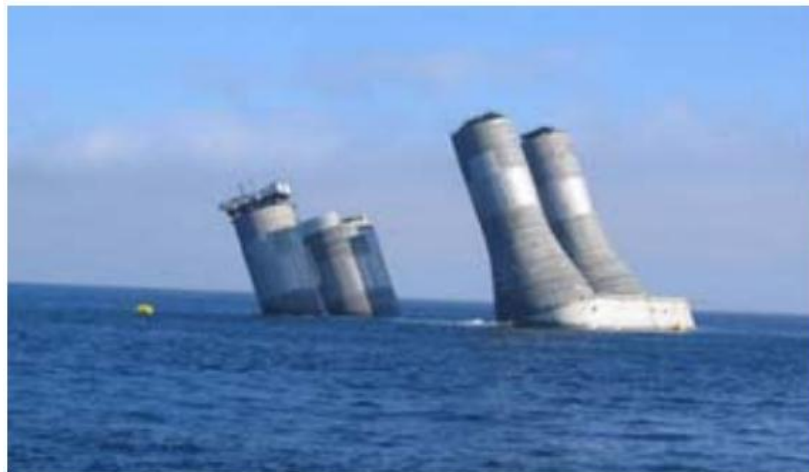
Figure 29: Inclined installation method in Sakhlin 2 (Vinci Ventus, 2010)
