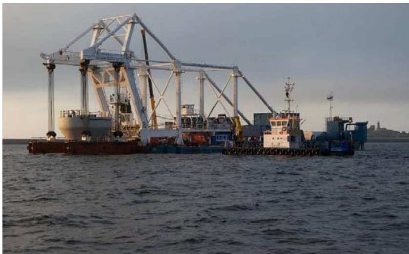
Figure 41: Foundation installation in Sprogø (ABJV, 2009)
