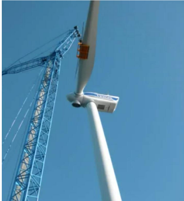
Turbine installation (ABJV)
