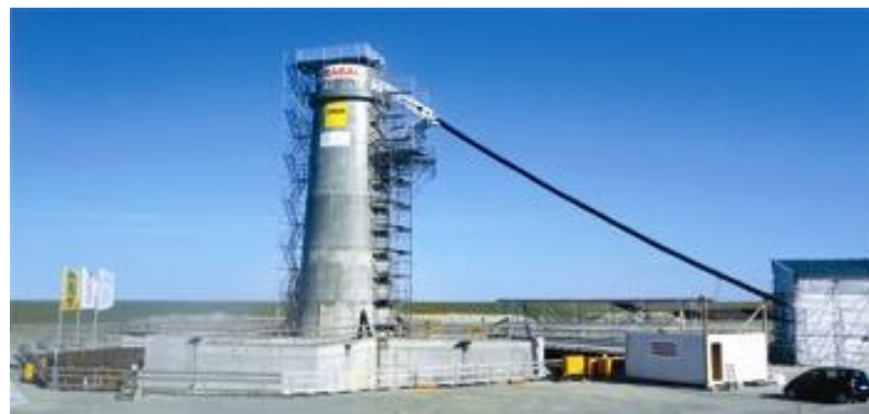
Foundation manufacture (Strabag)
