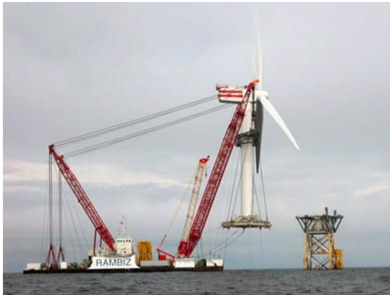
Figure 42: Pre-assembled turbine being installed in a jacket foundation (turbineel.net, 2013)
