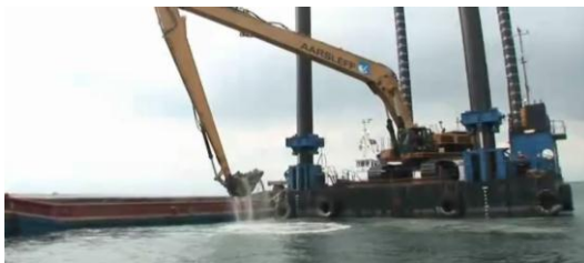
Seabed preparation (ABJV)
