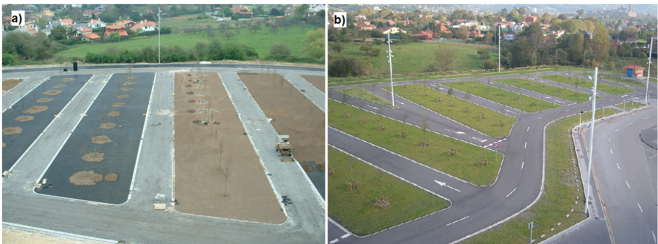
Figure 16. La Guia car park [71]. (a) Construction Phase; (b) Final Result.
