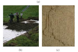
FIGURE 15: Geotextile equipped with the Fiber-ware special sensing cable and the Nexans standard indoor cable (yellow). Installation in two independent scenarios: the surface of a dike foot (b) and in a soil displacement (courtesy of K. Krebber).
