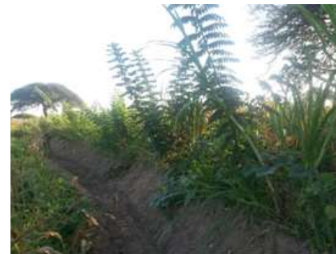
Stabilising erosion bunds
