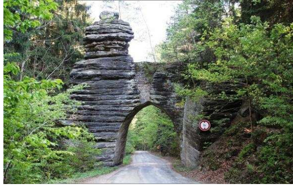
Fig. 4 Tunnel called Pekař's Gate – length 4 m
