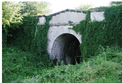
Fig. 1 Abandoned tunnel Slavíč
