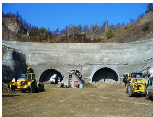
Fig. 5 South portal of the Prackovice tunnel
