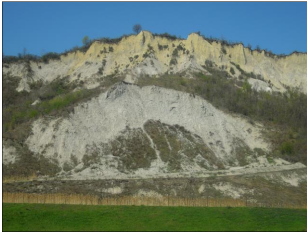
Figure 2 Argille Azzurre Formation (FAA) cropping out on the left-hand slope of the T. Corlo upper valley. In the top part of the cliff, ochre coloured sand layers are visible.
