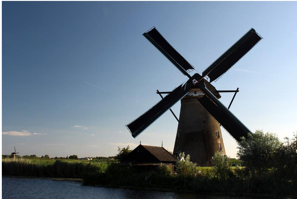
Figure 3: Wind mills used for drainage, reprinted from (Katicaj, 2016).
