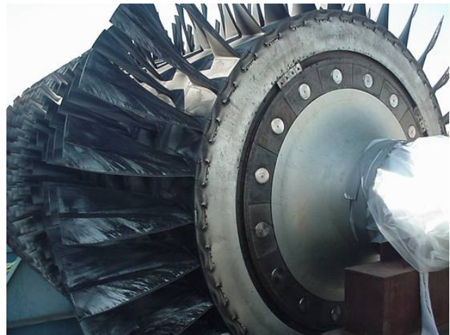
Figure 20: Oily Deposits on Axial Compressor Blades from No. 1 Bearing Oil Leakage on a Large Heavy Duty Gas Turbine
