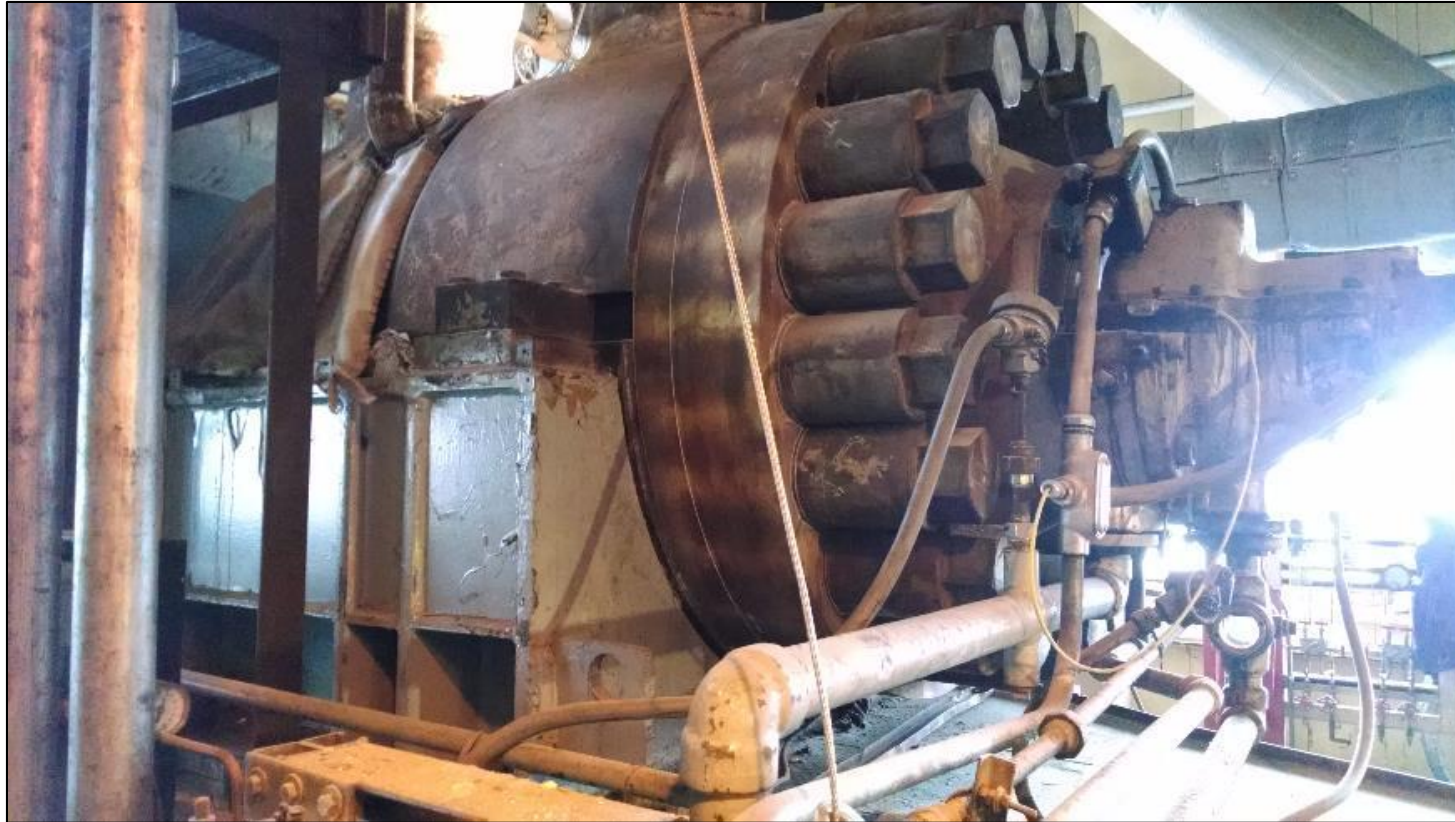
Viewed from north
