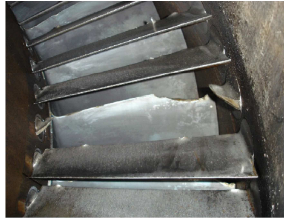
Figure 14: DOD Failure Relative to IGV (Inlet Guide Vane) Breakdown in the Axial Compressor.
