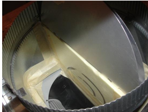
Figure 22: Airflow Guide Applied to Damper Outlet (Code: EXG)
